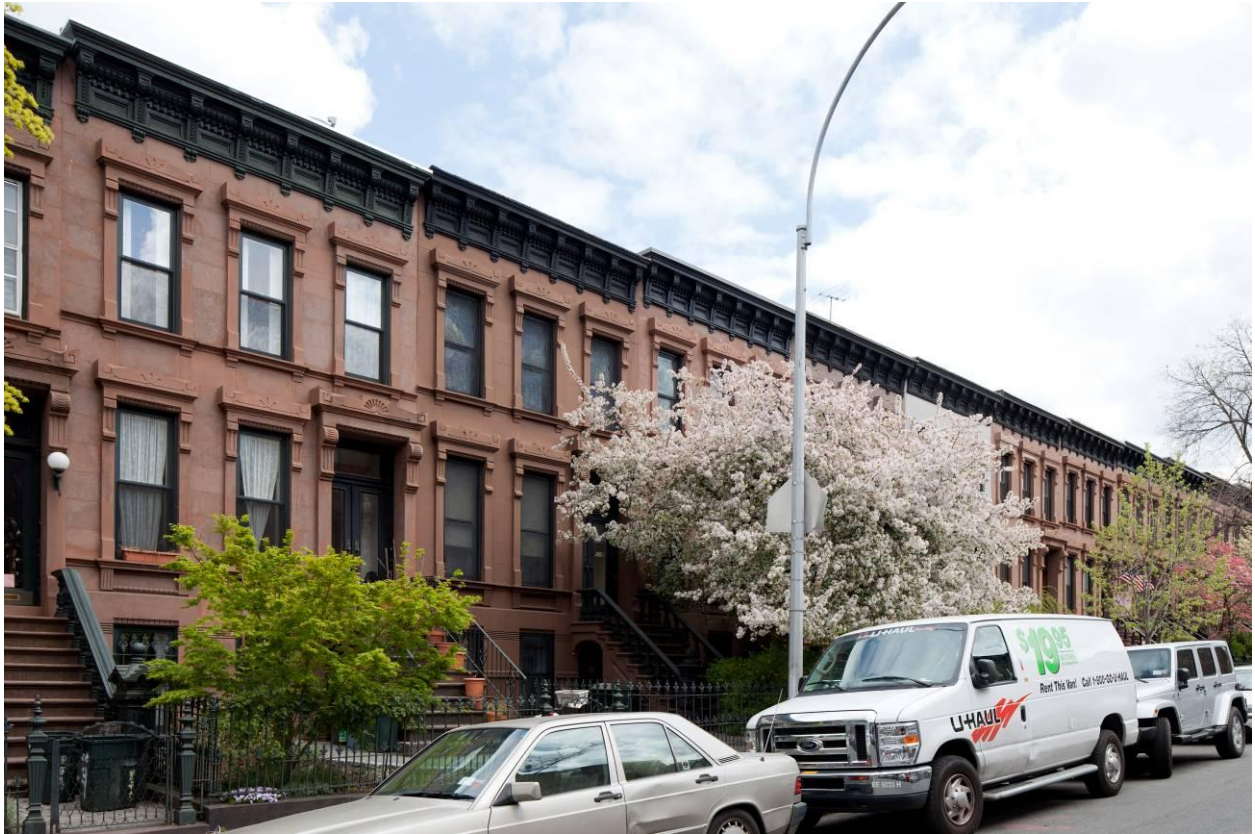
Figure 9 433 to 461 8 th Street Jefferson F. Wood, c. 1884 Photo: Christopher D. Brazee, 2012
