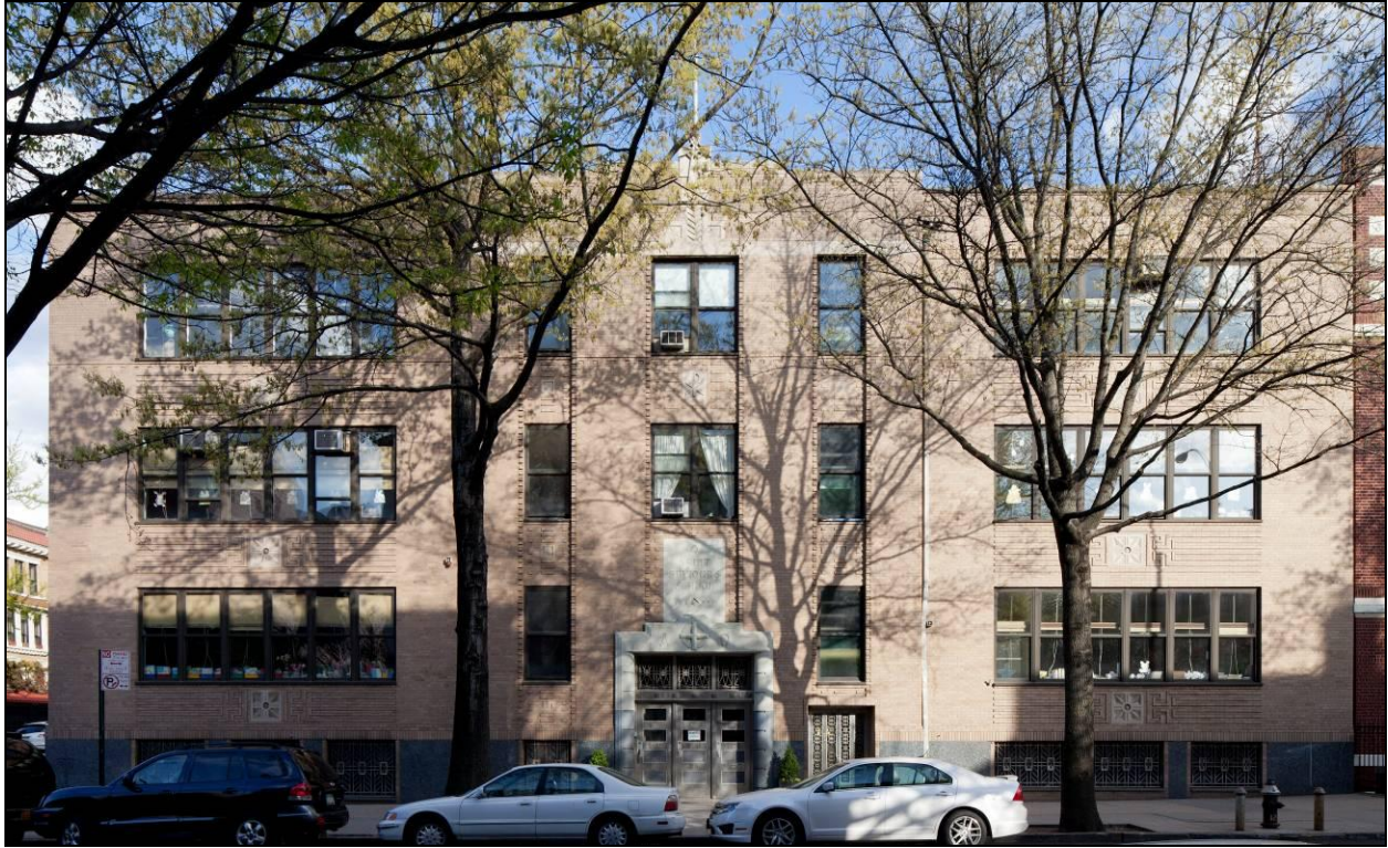
Figure 43 St. Saviour's School, 703 8 th Avenue Joseph Mathieu, c. 1955 Photo: Christopher D. Brazee, 2012
