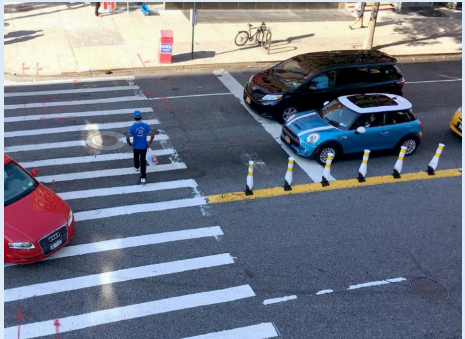
Right: Hardened centerline - rubber curb with delineators on the double yellow centerline.
