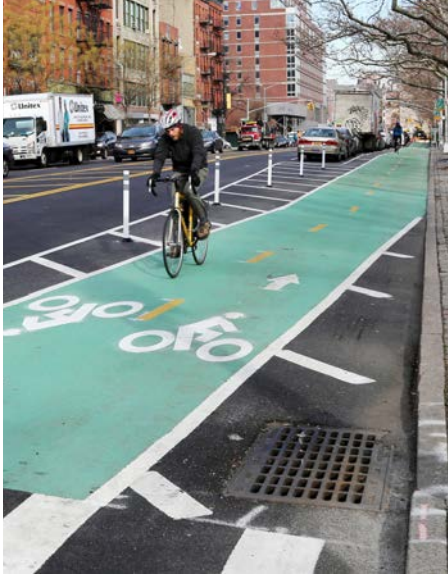
Chrystie Street protected bike lane.
