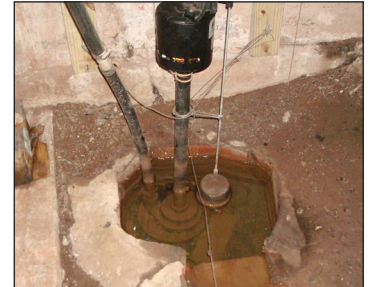
An illegal sump pump connected to the sewer system.
