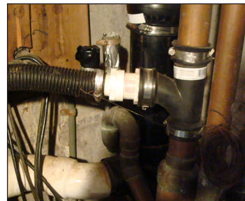
Illegal connection to the sewer system.
