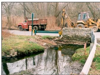
**Now:** The culvert was redesigned to abate flooding and to enhance aquatic habitat. Stones are placed in the streambed and through the culvert to provide habitat for aquatic life, and to attenuate the velocity of the water. Bluebelt field management staff keeps the culvert clear of sediment accumulations.
