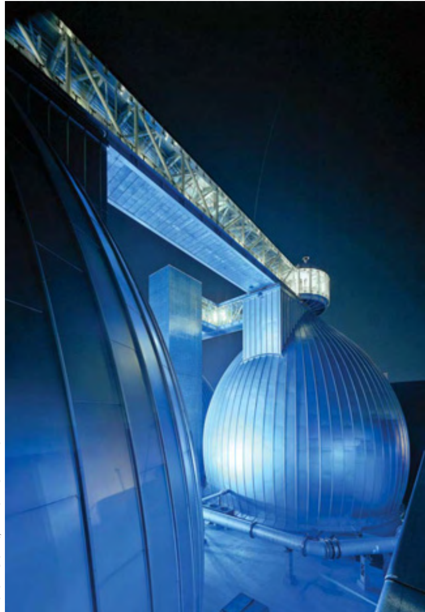
PHOTO: DIGESTERS, NEWTOWN CREEK WASTEWATER TREATMENT PLANT
