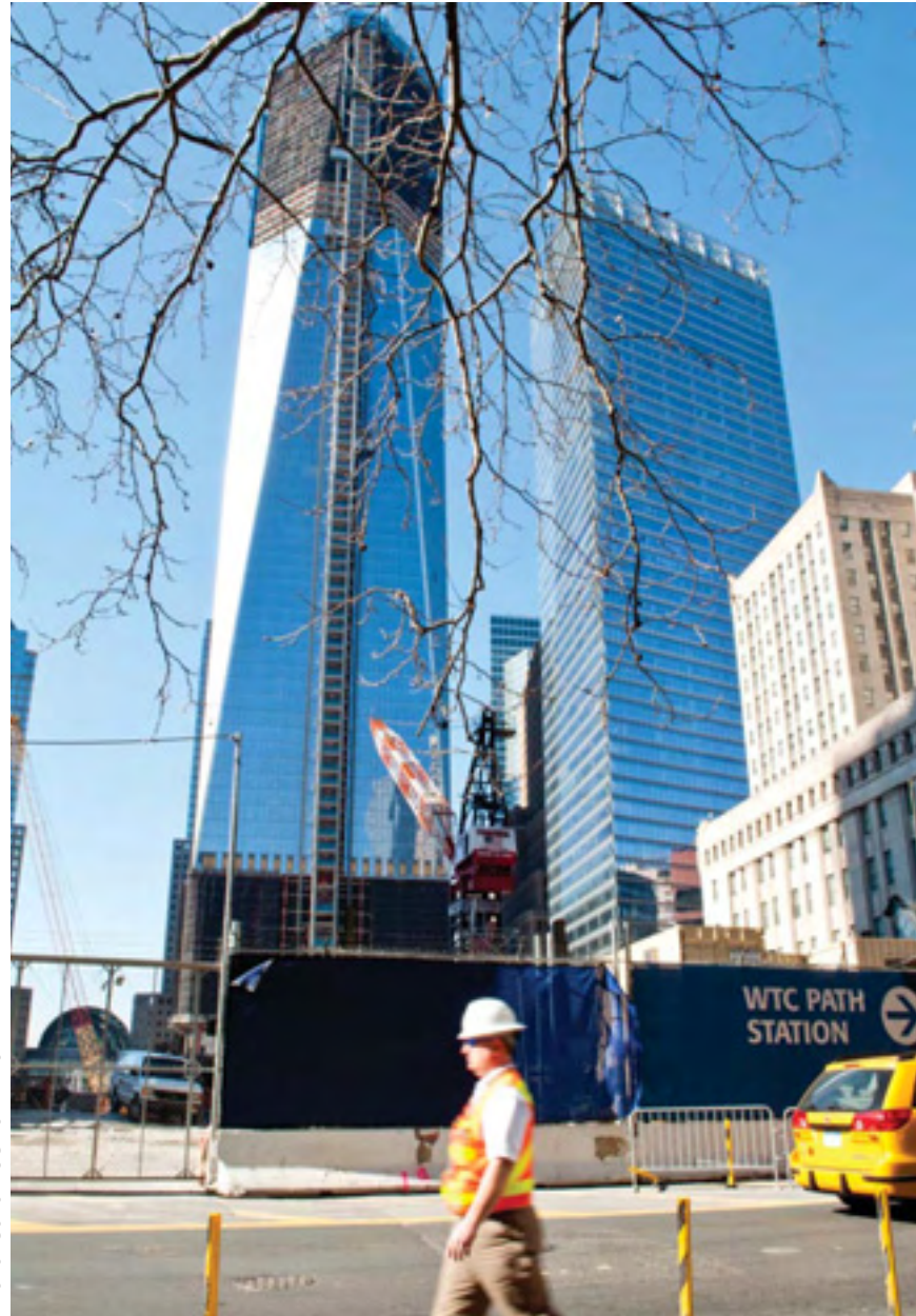
PHOTO: CONSTRUCTION IN LOWER MANHATTAN
