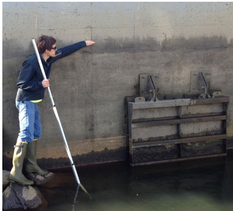
Geosyntec staff assessing tide gate condition and high water marks.
