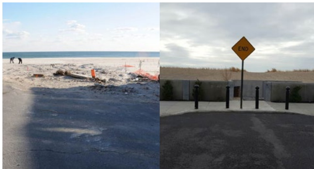
Before and after images of the Beach 133rd street end project in Belle Harbor, Queens, which included dune restoration, a concrete wall for added protection, sidewalk improvements, and landscaping.
