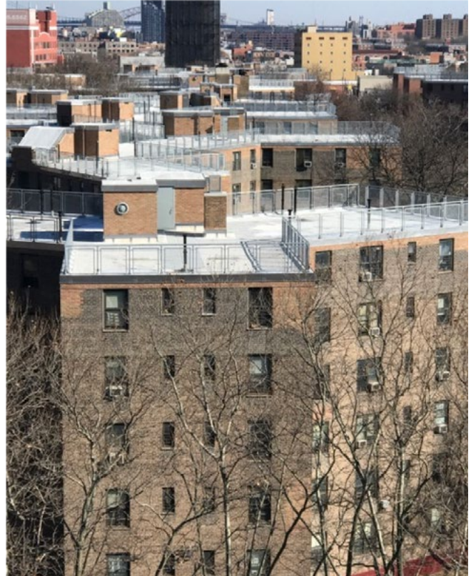
Newly replaced roofs at Queensbridge Houses
