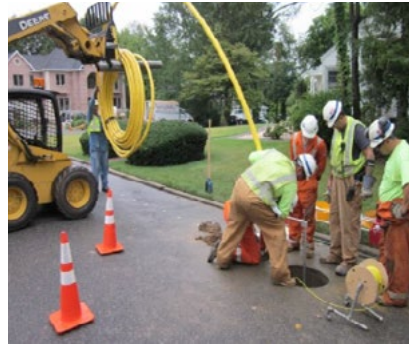
Workers with National Grid installing new infrastructure.
