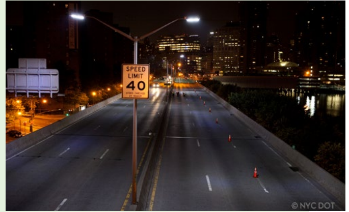
LED Streetlights on FDR Drive
