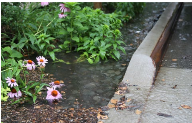
A curbside rain garden, part of the City's green infrastructure program, absorbs stormwater off streets and sidewalks during a rain event
