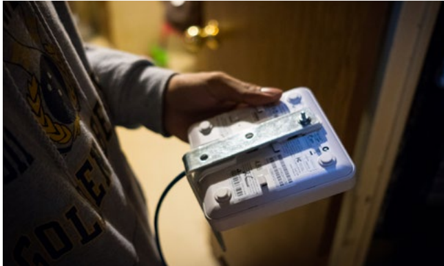
Quan holds a wireless router before installing in a closet.
