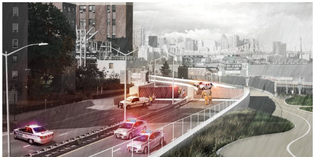
FDR Drive gate crossing with gates closing in preparation for a coastal flooding event.
