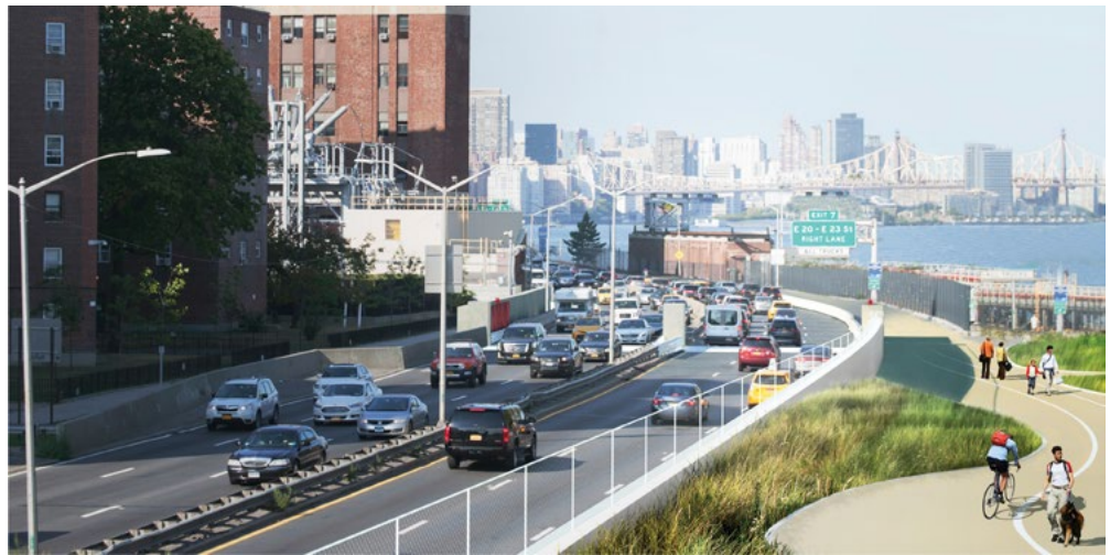
FDR Drive gate crossing with gates stored.
