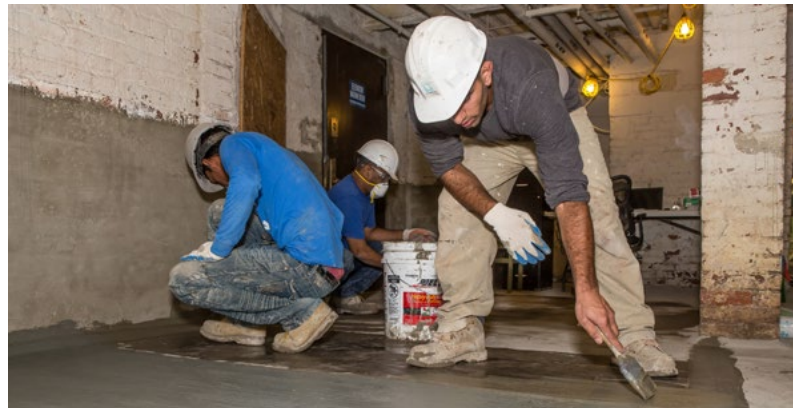
Waterproofing a basement floor
