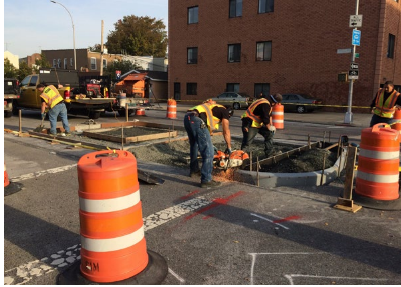
Constructing the Hoyt Avenue North protected bike lane in Queens
