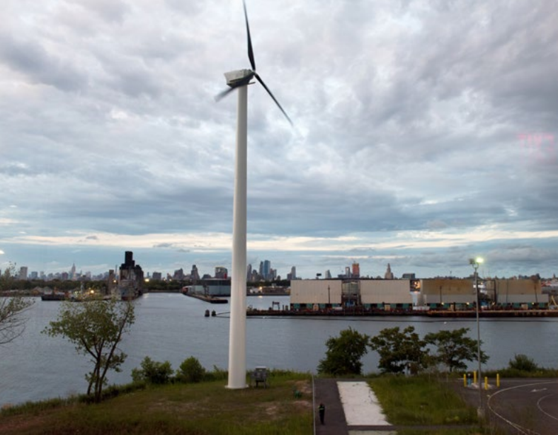
A commercial wind turbine on the Sunset Park Waterfront
