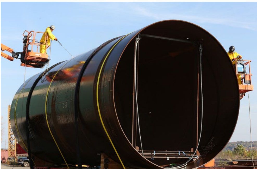
Steel liner for Kensico water tunnel
