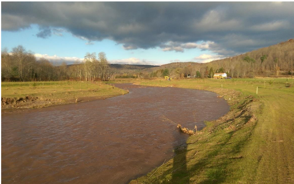
Figure 4.12 Batavia Kill at the Kastanis reach after construction
