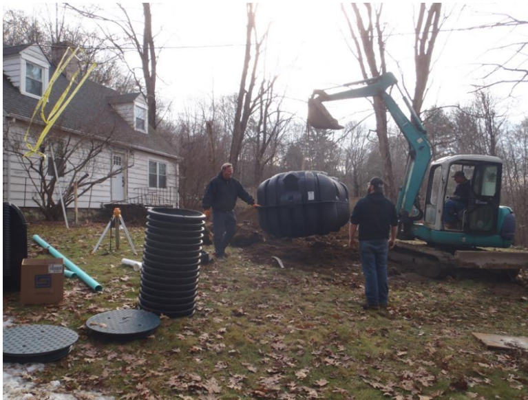
Figure 4.19 Septic tank replacement at a home in Kent in Putnam County.
