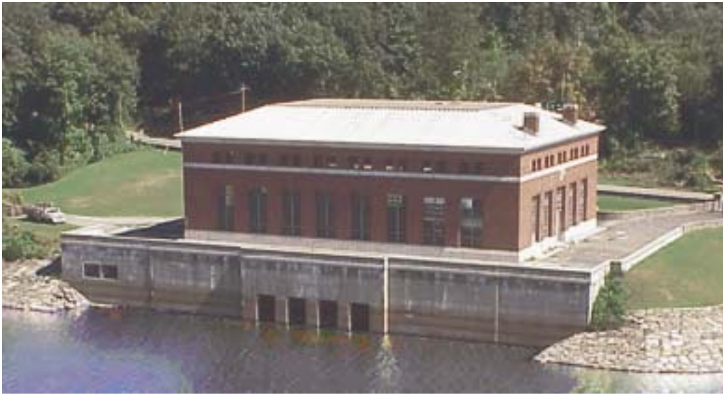
Figure 3.2 West Branch Reservoir upper intakes.
