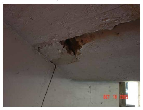
**BAYSIDE** Broken and crumbling concrete by the tactile strip on the eastbound platform. Observed: October 18, 2005.
