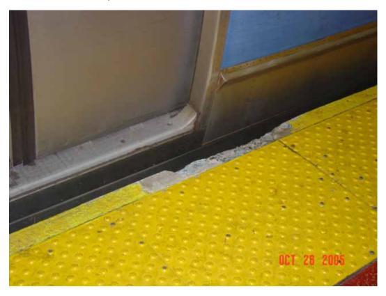
**PENN STATION** Exposed wiring at the edge of the Track 17 platform. Observed: October 26, 2005.
