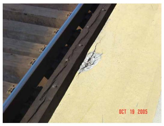
**PENN STATION** Broken concrete at the edge of the Track 19 platform. Observed: October 26, 2005.
