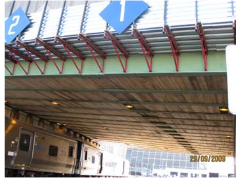
Installed Railroad Protective Shields.
