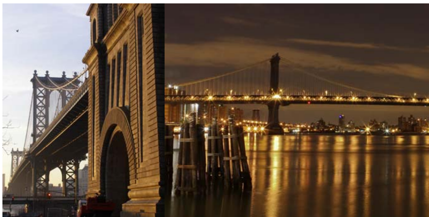
Manhattan Bridge. (Credit: Bojidar Yanev) Bridge at Night in May 2008. (Credit: Jason Bax)
