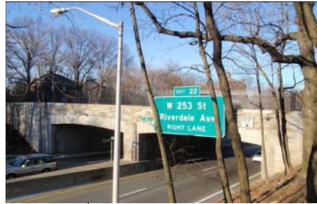
West 252 nd Street Bridge With New Signage.
