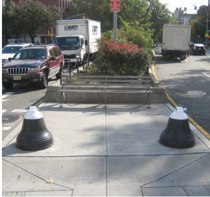
The project enhanced the median landscaping and provided seating where appropriate
