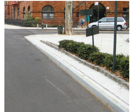
ABOVE: Typical untinted concrete curb with steel facing: West 114th Street and Morningside Avenue, Manhattan
