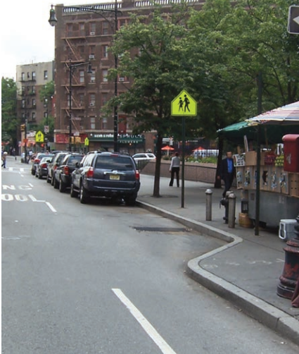
ABOVE: Curb extension: Seventh Avenue, Manhattan
