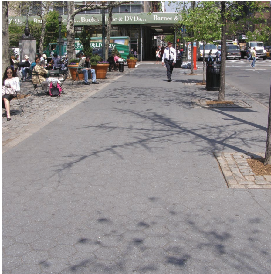
Hexagonal asphalt paver sidewalk: Columbus Avenue at West 66th Street, Manhattan
