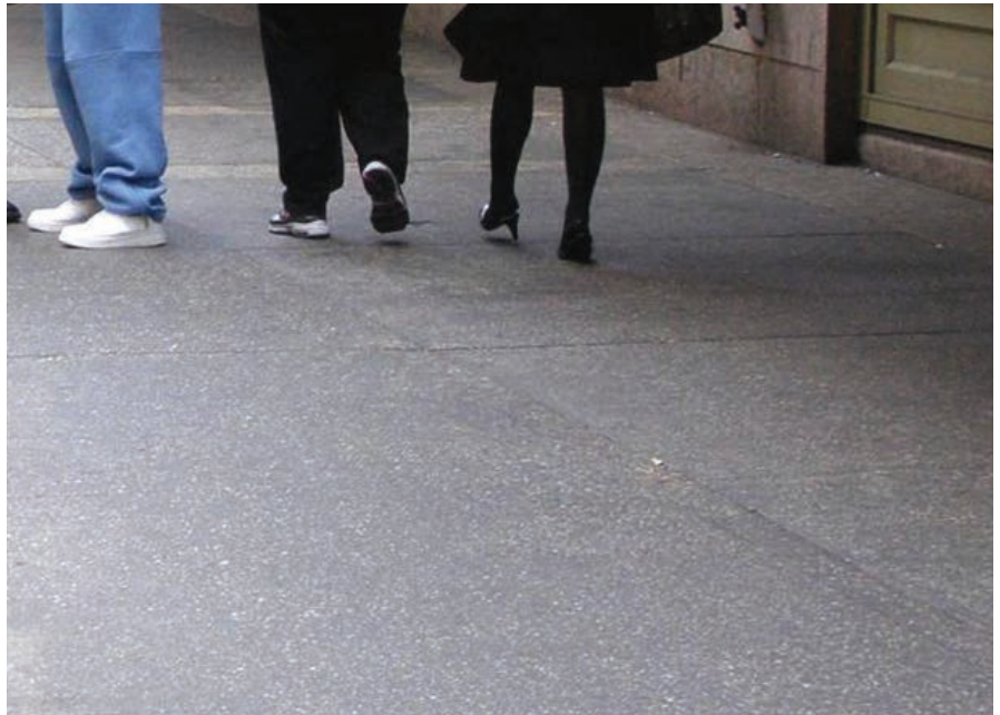
Tinted concrete sidewalk with light-colored exposed aggregate (note: this example does not include the required "simulated saw-cut joint" scoring pattern); East 42nd Street at Grand Central Terminal, Manhattan
