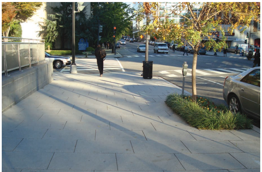
Concrete with London paver scoring: Washington, DC
