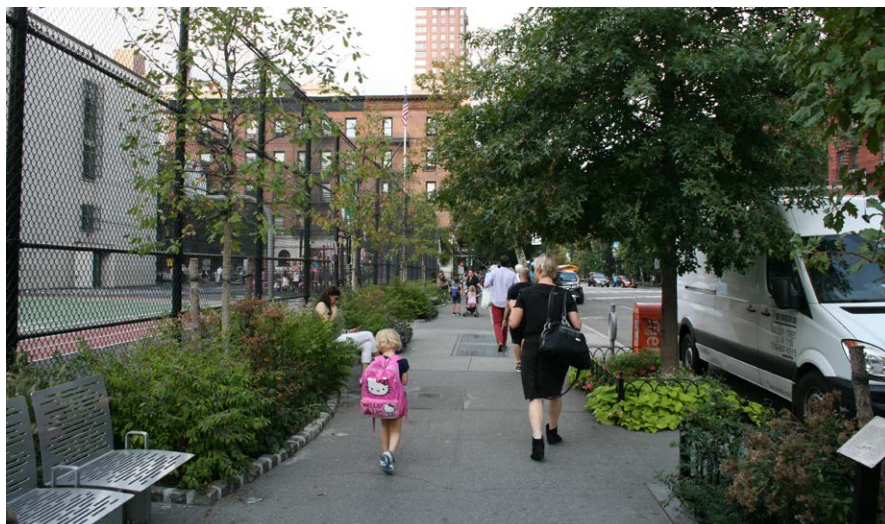
Streetscape enhancements on Columbus Avenue between West 76th and 77th Streets included CityBenches, planting areas bounded by reused granite pavers, and new tree-bed guards: Manhattan
