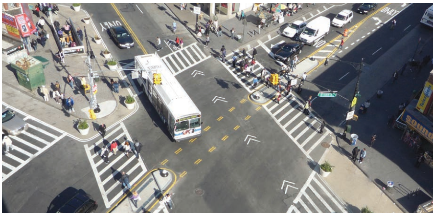
DOT upgraded the complex intersection of Melrose Avenue, Third Avenue, and East 149th Street — known as the Hub — in 2008. Bronx
