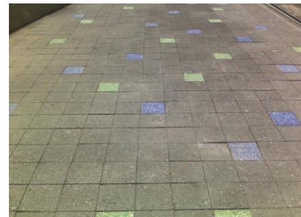
Concrete pavers with exposed blue and green glass aggregate (shown interspersed with black asphalt pavers): Hudson River Park, Manhattan
