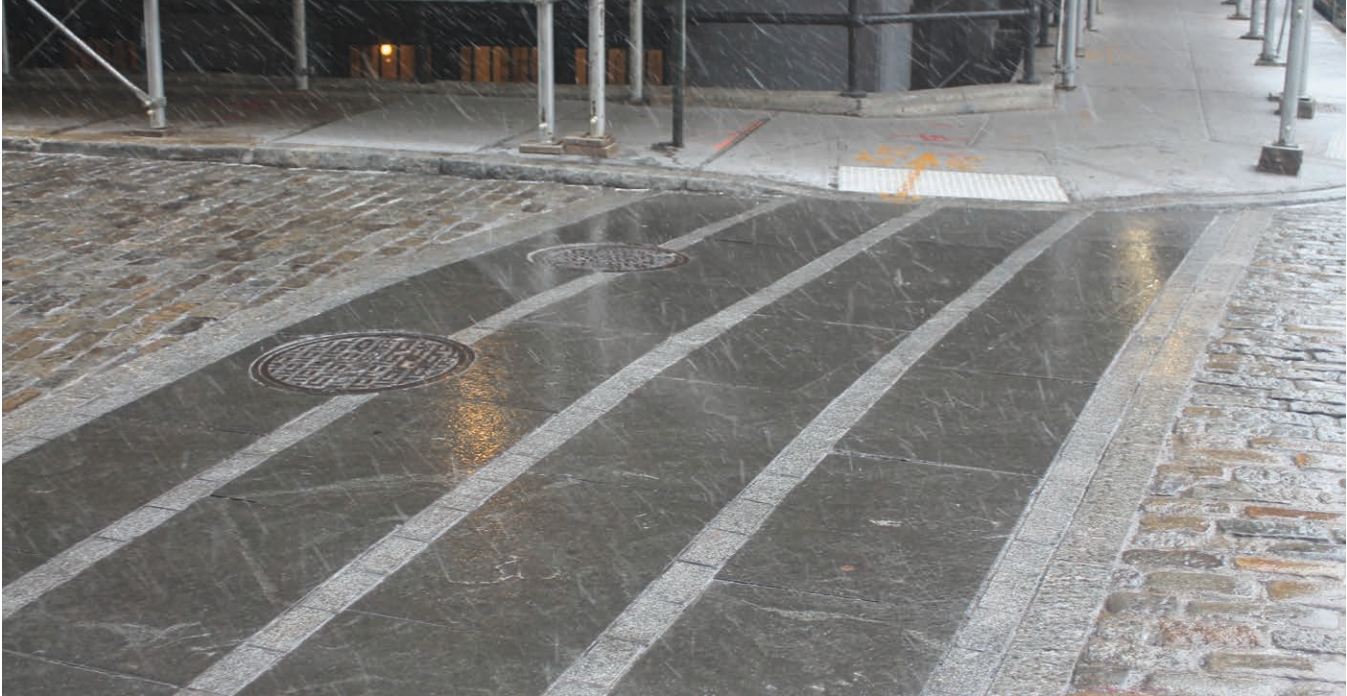
Granite pavers in a crosswalk. This treatment is appropriate for historic districts: Water Street, Brooklyn
