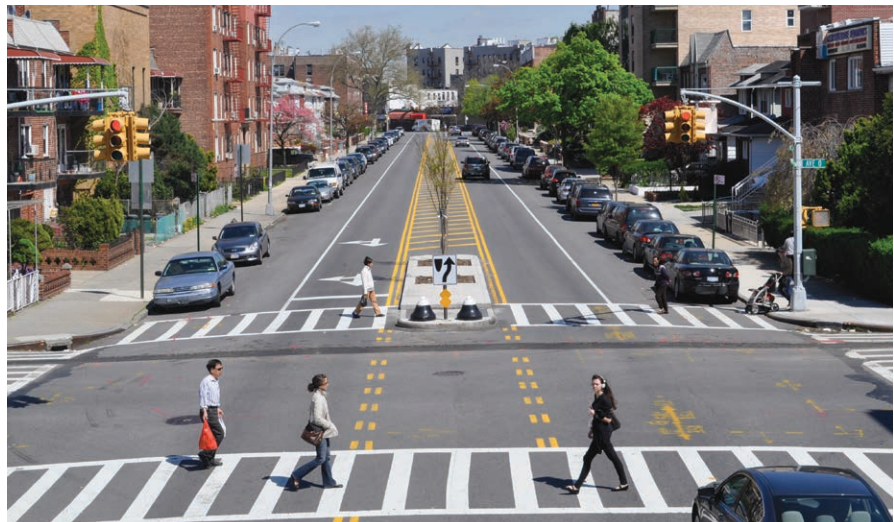
After: DOT installed a "road diet" in 2010, resulting in a 25% reduction in crashes
