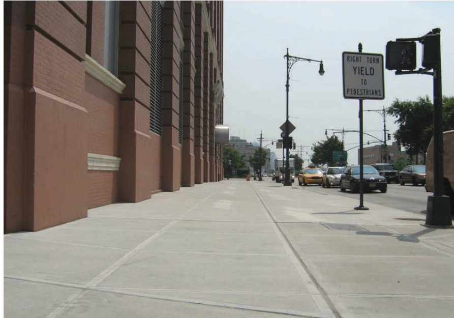
Sidewalk with standard paving treatment: 11th Avenue, Manhattan
