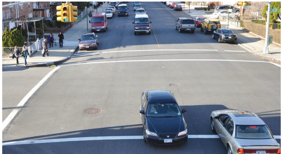
Before: After two fatalities occurred at the same intersection in one year, DOT found that the roadway was over capacity: West 6th Street, Brooklyn
