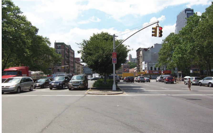
Typical asphalt roadway: Delancey Street at Forsyth Street, Manhattan
