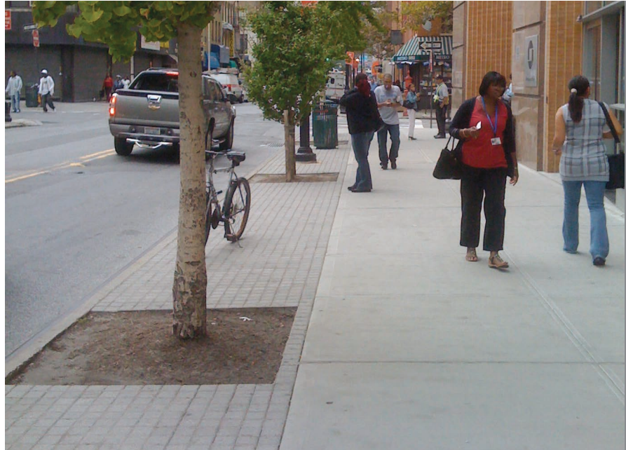
Square asphalt pavers in a furnishing zone: Willoughby Street at Duffield Street, Brooklyn
