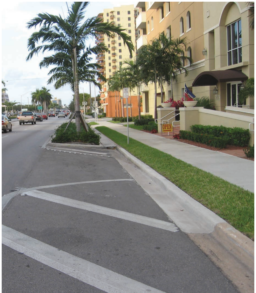
Precast concrete curb and gutter sections laid end-to-end. Photo shows extension in background: Miami Beach, FL (Note: for illustrative purposes only)
