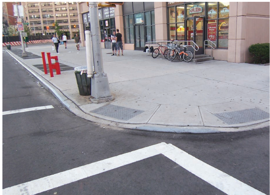
Sidewalk corner with pedestrian ramps: West 110th Street, Manhattan
