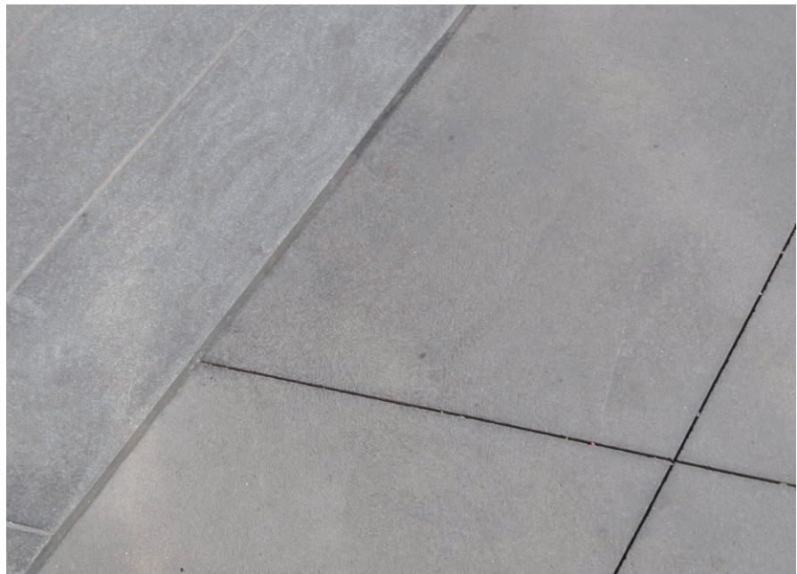
Concrete pigmented to match adjacent granite: Greenwich Street at Barclay Street, Manhattan
