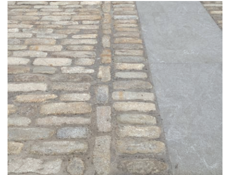
Detail of a design to provide rideable cycling surface using a strip of smooth granite pavers among reused granite blocks
