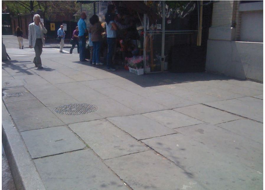
Bluestone pavers in the foreground and concrete pigmented to simulate the historic pavers in the background: Hudson Street at Christopher Street, Manhattan
