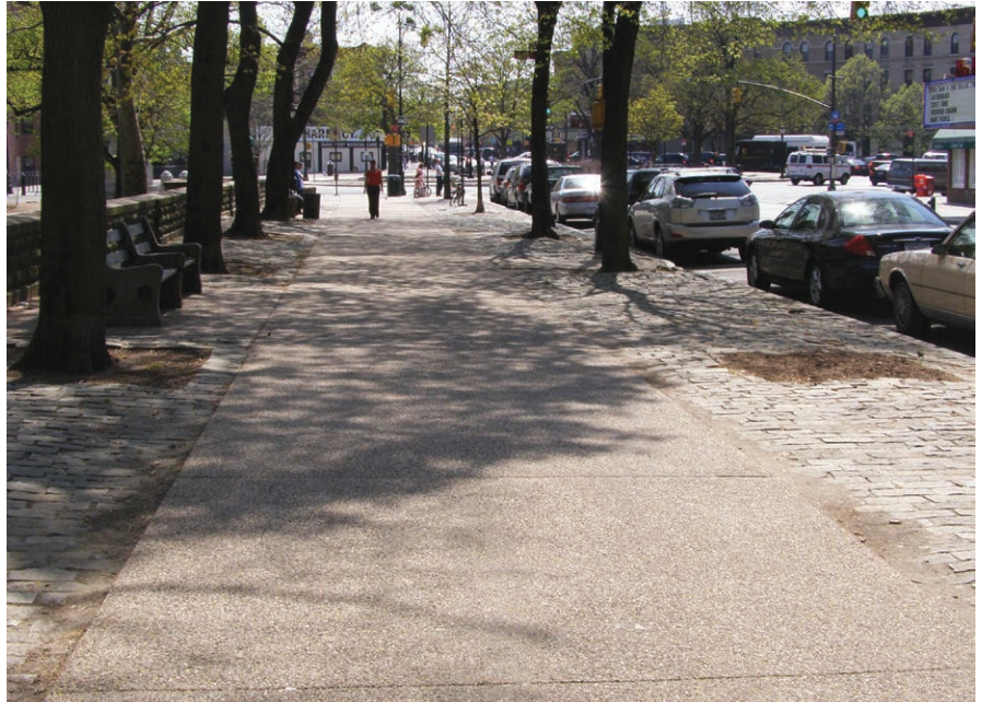
Sand-colored concrete sidewalk with exposed aggregate: Prospect Park West, Brooklyn
