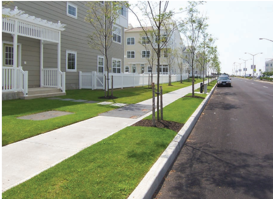
ABOVE: Typical untinted concrete curb with steel facing: West 114th Street and Morningside Avenue, Manhattan
