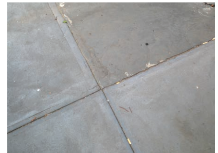
Concrete pigmented to simulate bluestone adjacent to a bluestone flag: Pacific Street, Brooklyn
