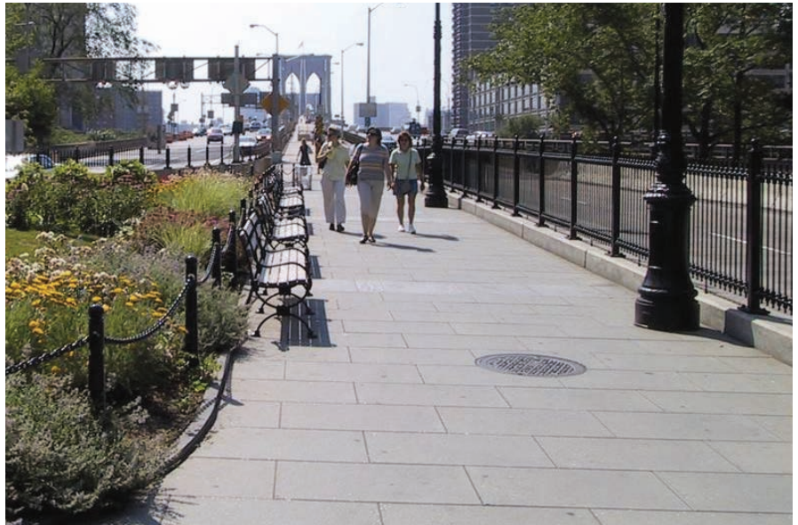
Concrete with London paver scoring: Brooklyn Bridge pedestrian access ramp, Manhattan
