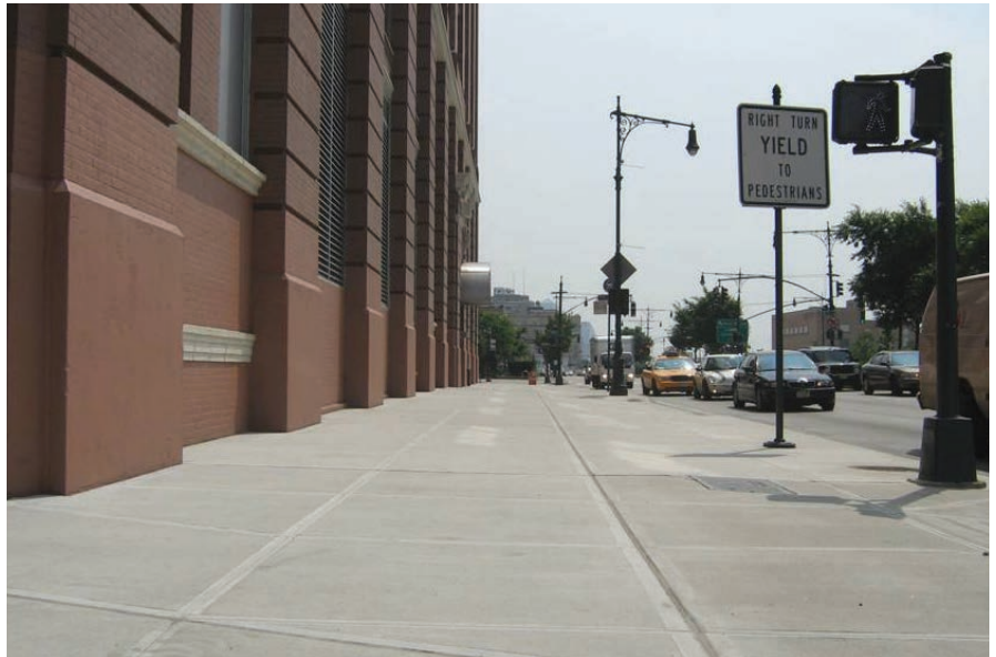
Typical concrete sidewalk: West Street at 16th Street, Manhattan
