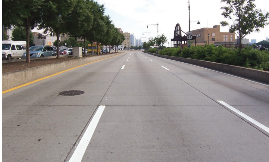
Typical concrete roadbed: West Side Highway, Manhattan
