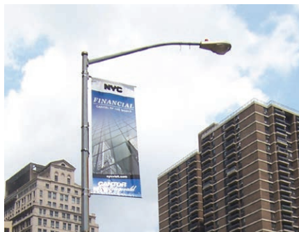
Cobra Head luminaire on Octagonal pole: Pearl Street, Manhattan
