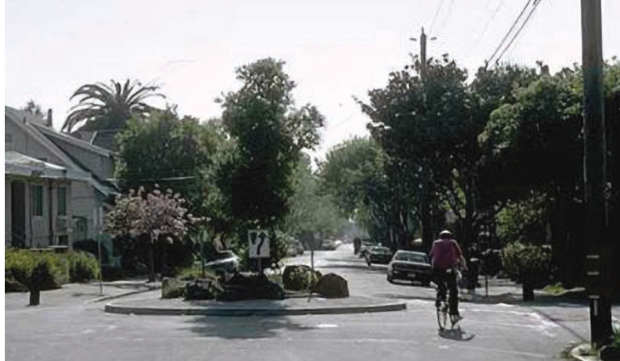
Neighborhood traffic circle with landscaping: Berkeley, California (Credit: John Allen) (Note: for illustrative purposes only)
