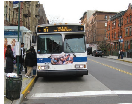
Typical concrete bus pad: Manhattan Avenue at 114th Street, Manhattan
