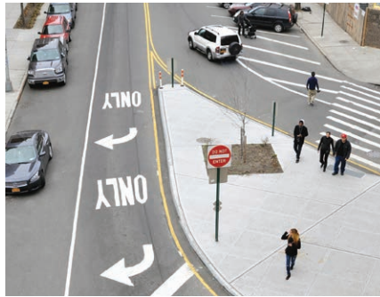
Operational safety enhancement: Louis Nine Boulevard, Bronx
