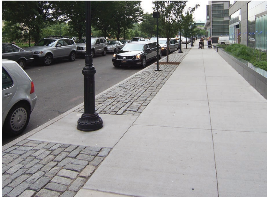
Granite blocks are for use in furnishing zones only: Little West Street, Battery Park City, Manhattan
