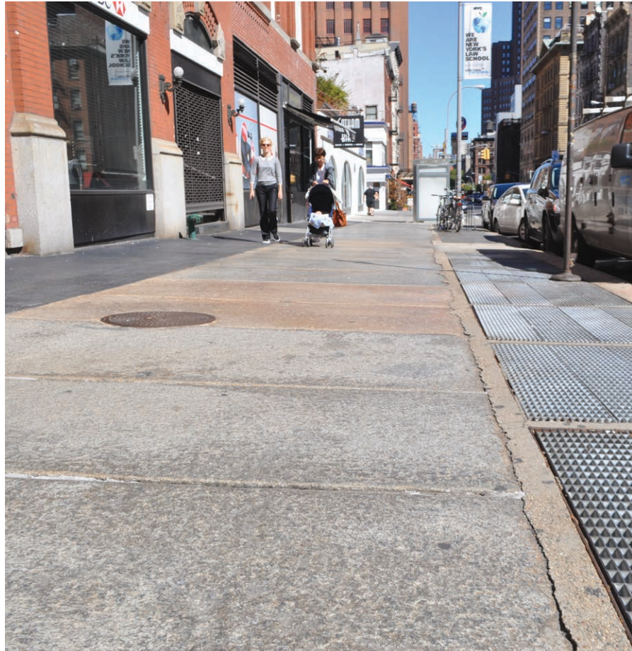
Granite slab sidewalk: West Broadway at Reade Street, Manhattan
