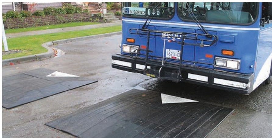
Speed cushions showing ease of bus passage: Vancouver, Canada (Credit: Richard Drdul) (Note: for illustrative purposes only)
