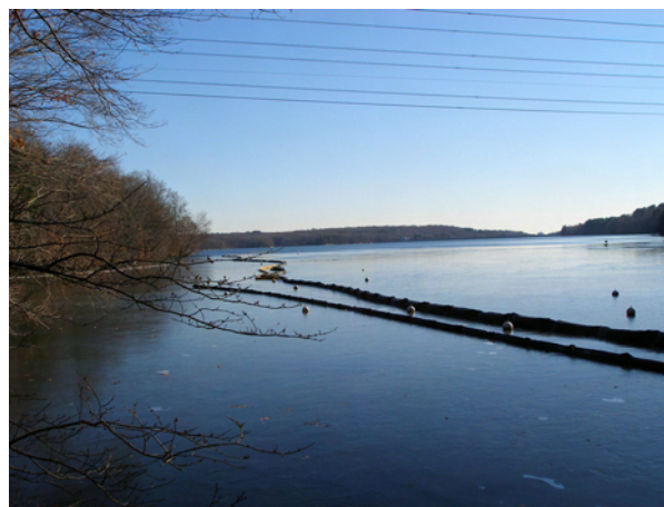
Figure 6.4 Photograph of turbidity curtain in the Catskill Upper Effluent Chamber cove.
