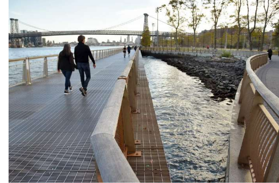
Separated Esplanade example at East River Park (Photo Credit: Nathan Kensinger)
