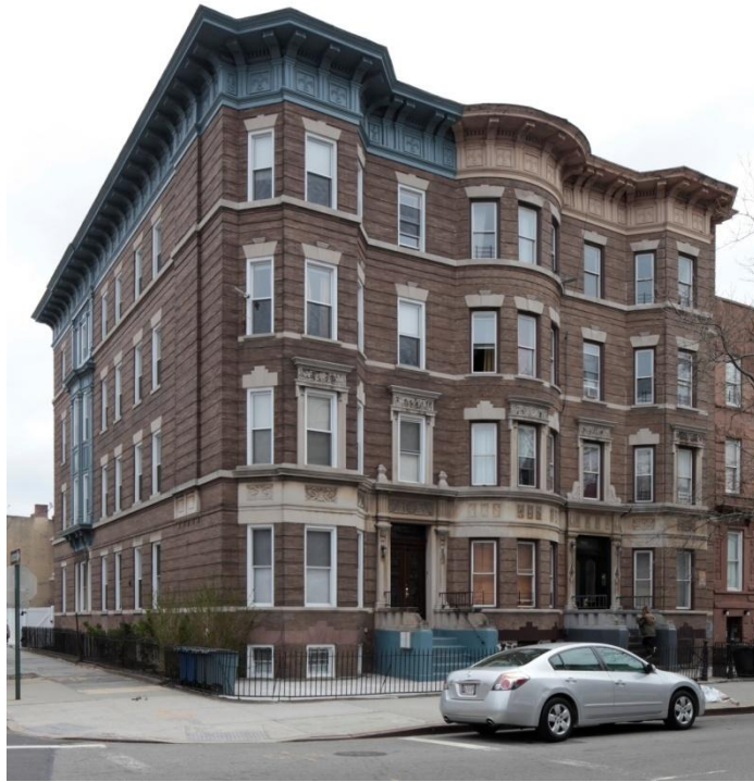
291 and 293 Stuyvesant Avenue (1898, Axel S. Hedman, architect): These Renaissance Revival style apartment houses feature full-height angled and round bays, decorative stoop parapets with buttresses, classical main-entrance surround featuring pilasters and foliate ornament, and molded cornices. Photo: Christopher D. Brazee, 2013
