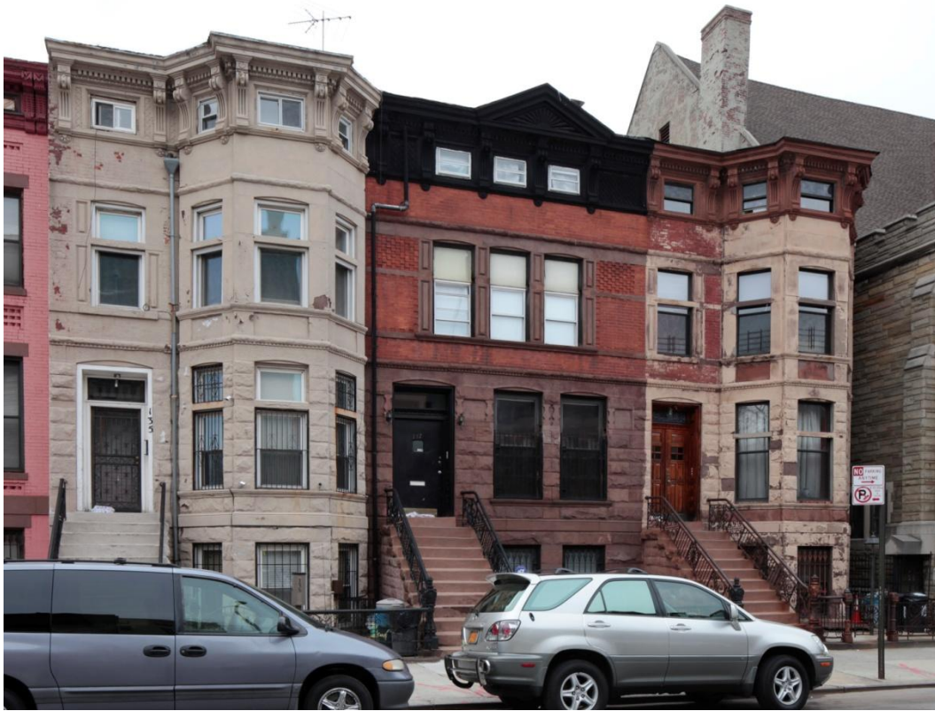
135 to 139 Decatur Street (1890, John L. Young, architect): This three-building, Queen Anne style row, arranged in an A-B-A pattern, features rough-faced brownstone ashlar, transom window sash above wide rails, and bracketed cornices topped by gables containing sunbursts. Photo: Christopher D. Brazee, 2013
