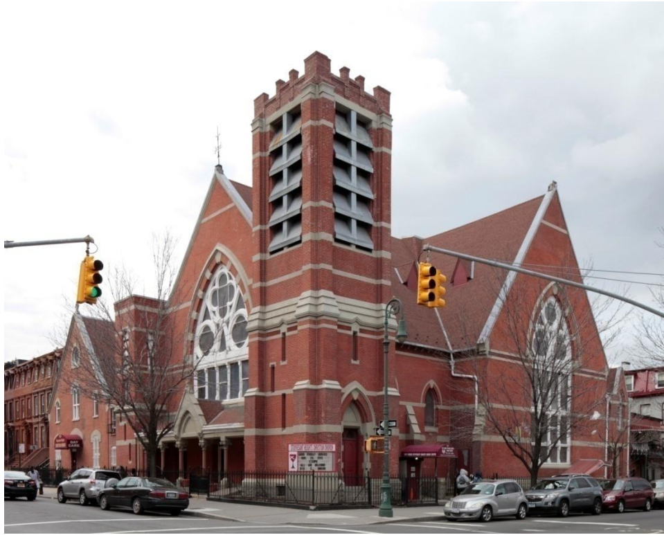
Tompkins Avenue Presbyterian Church (now the Stuyvesant Heights Christian Church) 61-73 Mac Donough Street (aka 458-468 Tompkins Avenue), built c.1873-74, was designed by architect George Hathorne in a simplified interpretation of the Victorian Gothic style. Photo: Christopher D. Brazee, 2013
