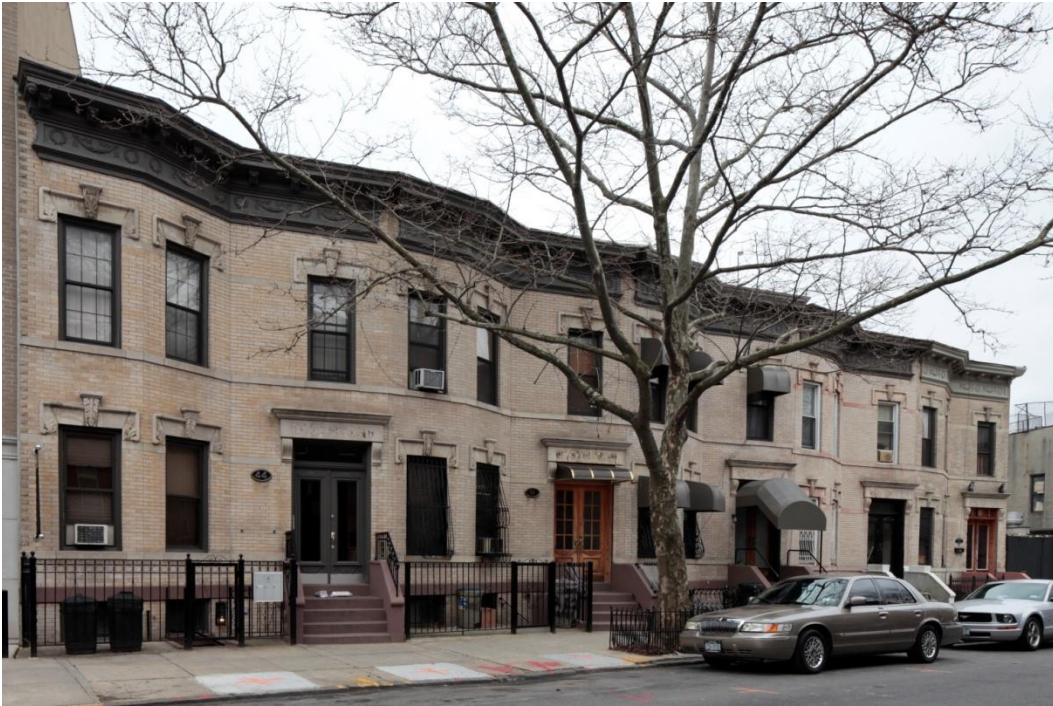
36 to 44 Decatur Street (1907, Louis Berger & Co., architects): Another row that mixes the two styles, these houses feature prominent Renaissance-inspired pressed-metal cornices decorated with swags, wreaths, scrolled modillions, and egg-and-dart moldings, as well as Romanesque-style foliated label lintels and keystones. Photo: Christopher D. Brazee, 2013
