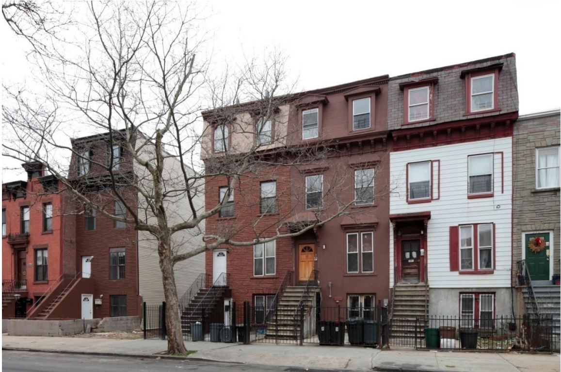
340 to 346A Decatur Street, a wood-frame, Second Empire style row (with alterations), built in 1873-75 when Bedford-Stuyvesant was being transformed from a suburb of farm fields and estates to a dense urban neighborhood. Photo: Christopher D. Brazee, 2013
