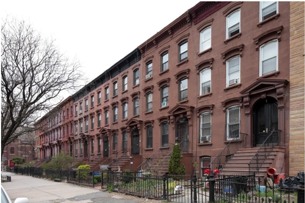
267 to 287 Macon Street , built in 1872-73, display typical characteristics of Italianate style row houses, such as pedimented door hoods supported by large scrolled brackets, segmentally-arched window openings with molded and bracketed lintels, and projecting cornices with frieze panels and dentils. Photo: Christopher D. Brazee, 2013
