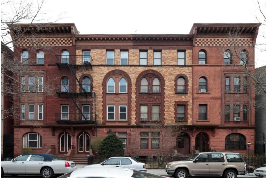
88 to 94 Decatur Street (1889, Sibell & Miller, architects): This short row forms an excellent example of the Romanesque Revival style as applied to row house design; the two end houses are mirror images of each, as are the two center buildings, thereby creating a symmetrically composed ensemble. Photo: Christopher D. Brazee, 2013
