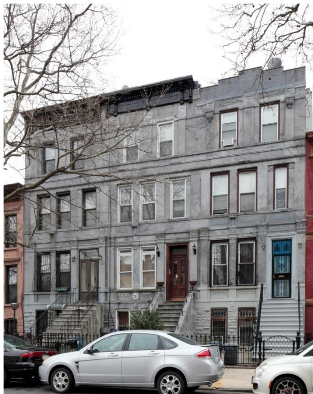
326 to 328 Decatur Street (1886, John C. Bushfield, architect): This unusual, marble-fronted trio of houses has Renaissance Revival style features, such as pilasters with carved capitals, scrolled and foliated brackets, paneled spandrels, and bracketed cornices with dentils. Photo: Christopher D. Brazee, 2013
