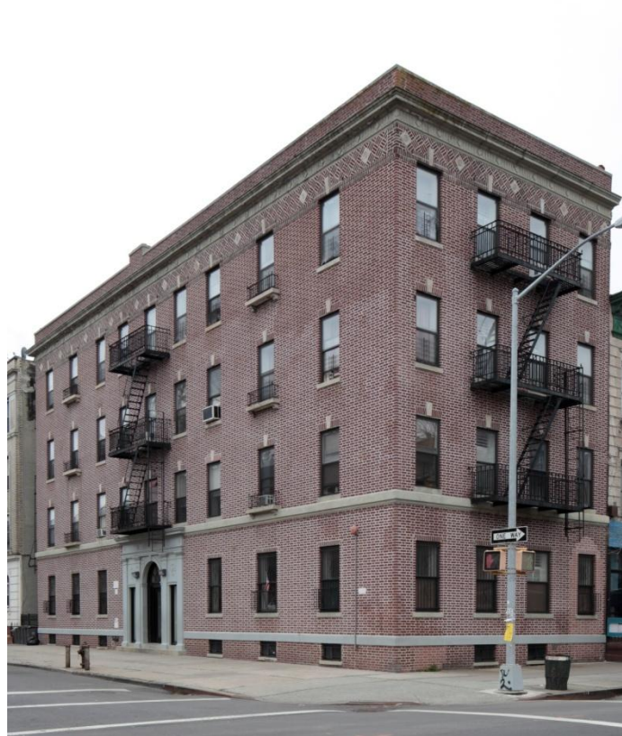
Library Court, 372 Lewis Avenue (aka 405-409 Macon Street) : Designed by architect W.T. McCarthy and built in 1914, this Colonial Revival style apartment house was probably given its name due to its location across the street from the Macon Branch of the Brooklyn Public Library. Photo: Christopher D. Brazee, 2013
