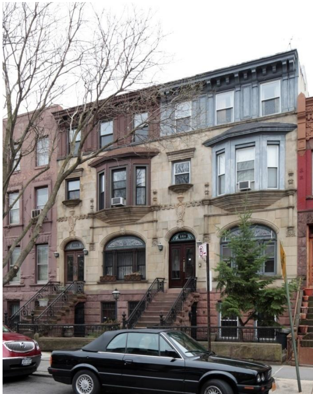
160 and 162 Bainbridge Street These unusual Chateausque style row houses, designed by Daniel B. Norris and built in 1892, feature elaborate façade detailing, such as cartouches, foliage, ribbonwork, and intricate moldings. Photo: Christopher D. Brazee, 2013
