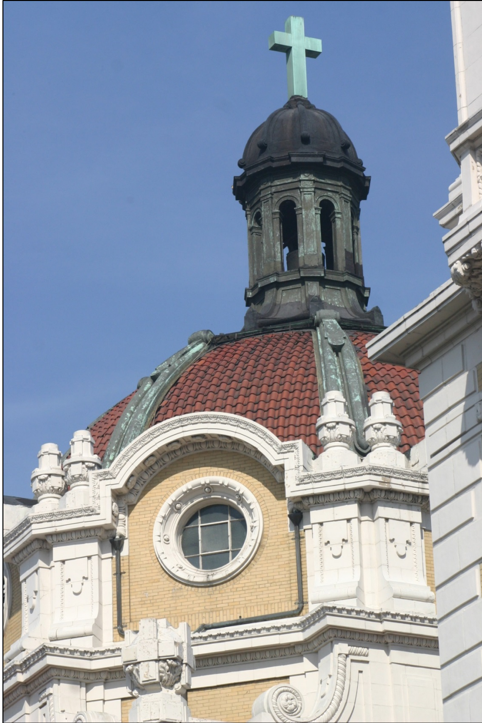
Saint Barbara's Roman Catholic Church Dome detail (Photo: Christopher D. Brazee, 2007)
