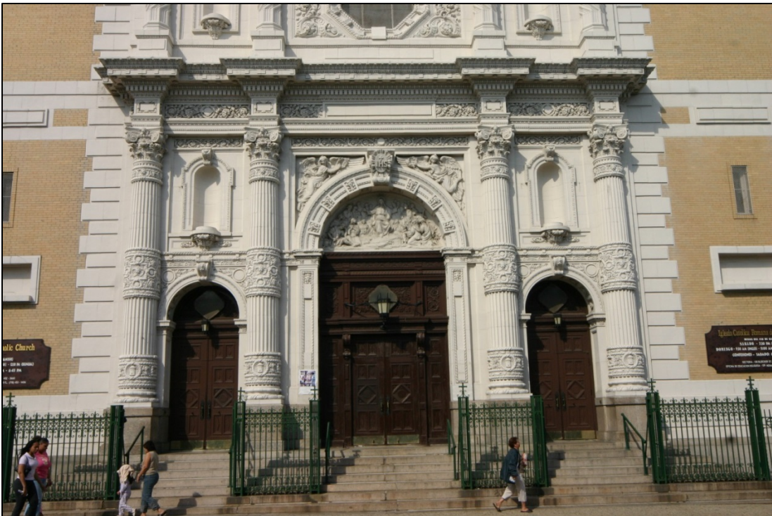
Saint Barbara's Roman Catholic Church Main facade details (Photo: Christopher D. Brazee, 2007)
