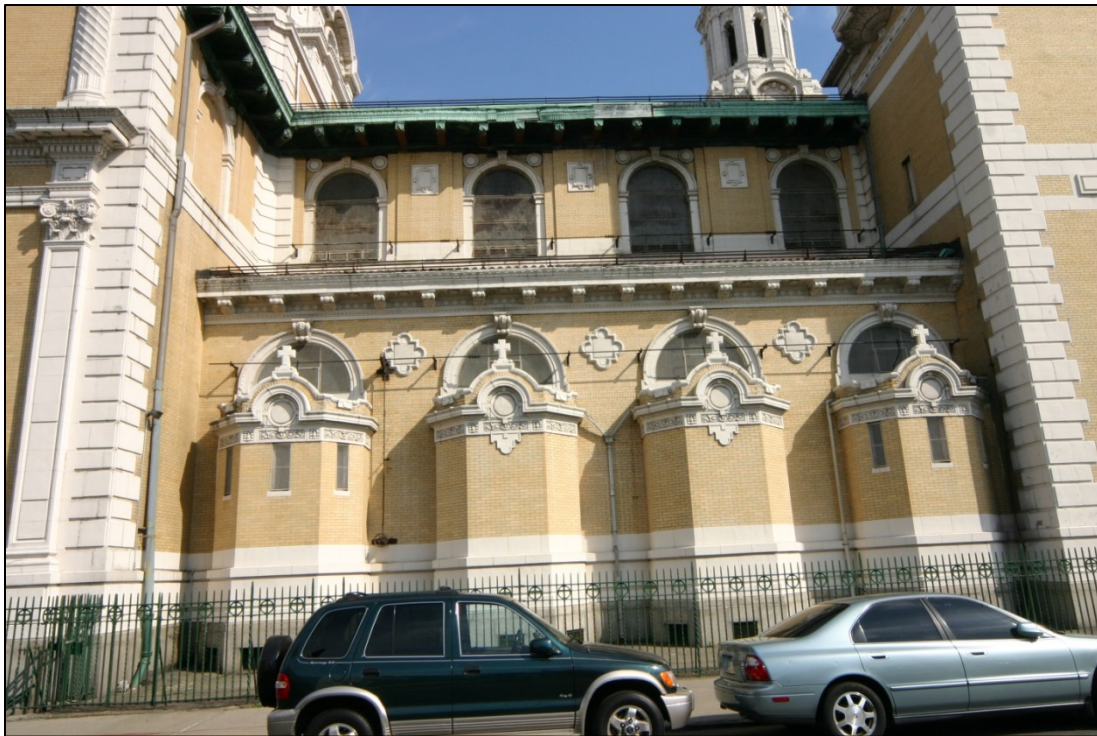
Saint Barbara's Roman Catholic Church Main facade details (Photo: Christopher D. Brazee, 2007)
