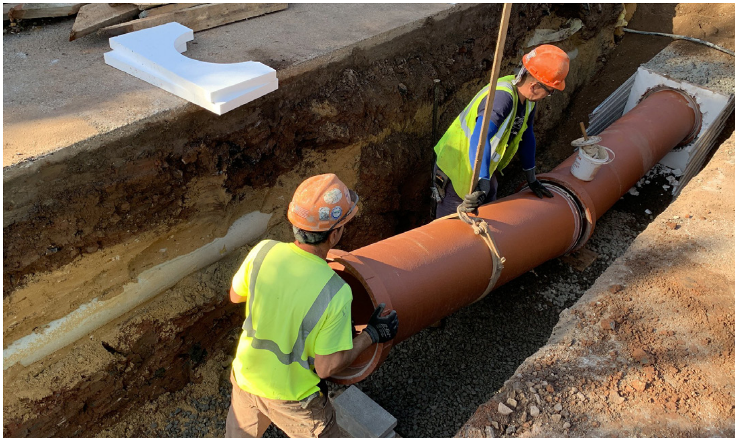
Installation of New Catch Basins for Willowbrook/Westerleigh
