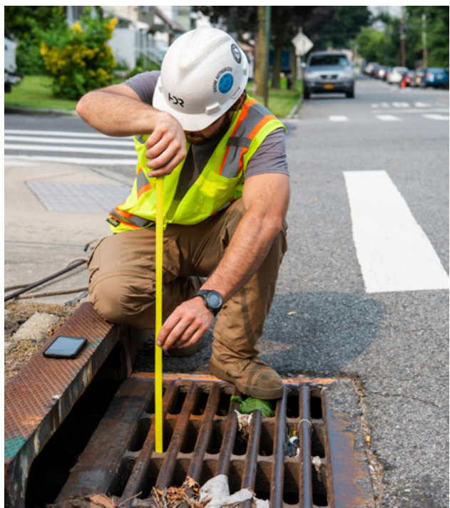
Measuring debris in catch basin for Loading Rate Study
