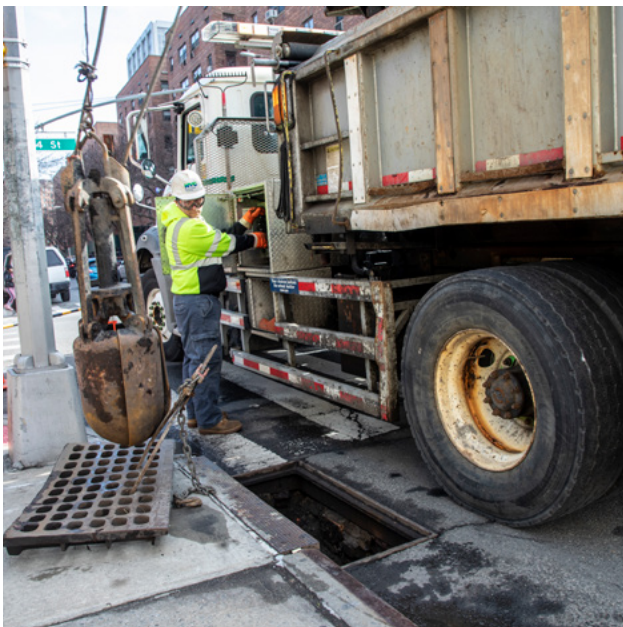
DEP catch basin cleaning
