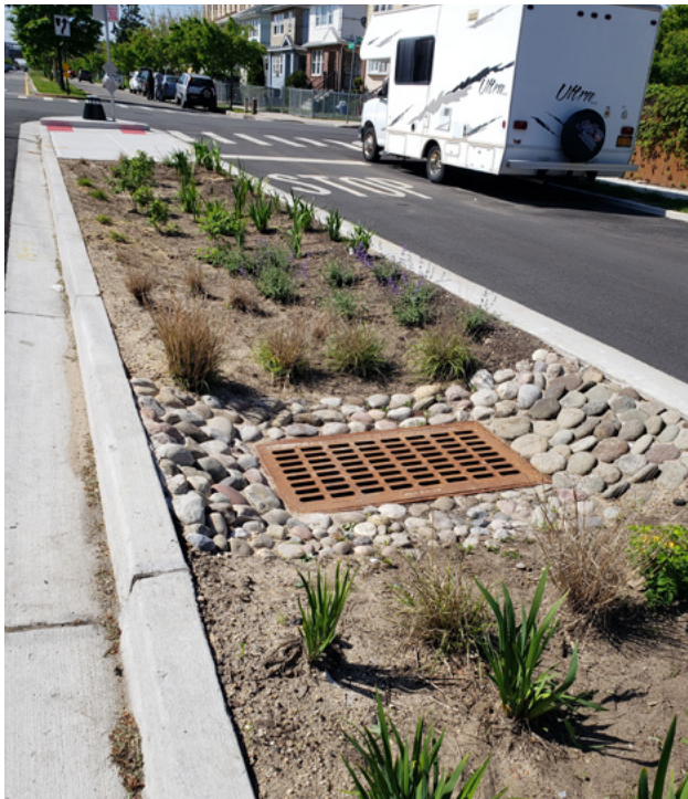
Rockaway Median Project
