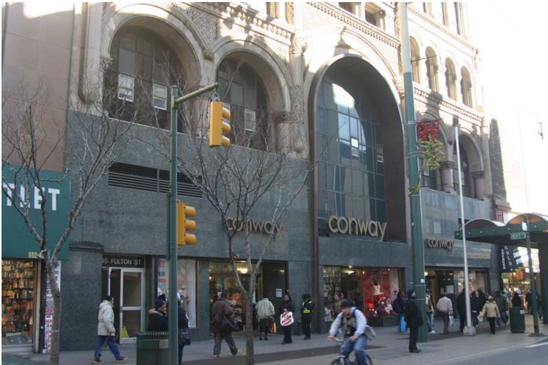
Offerman Building Fulton Street, details, lower floors and base Photos: Carl Forster
