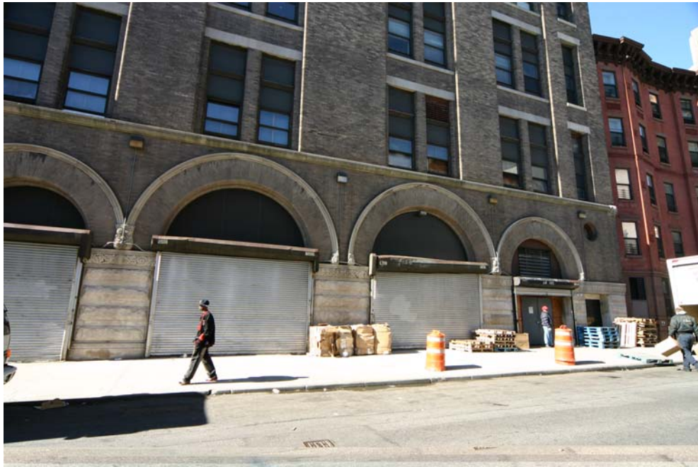
Offerman Building Duffield Street elevation Photos: Carl Forster
