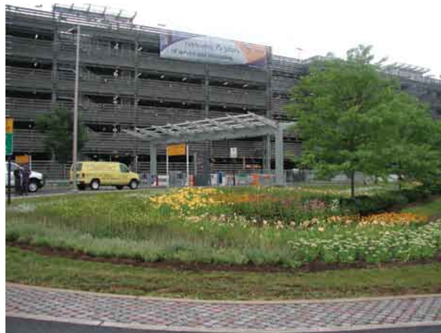
Newark Liberty International Airport infiltration trench
