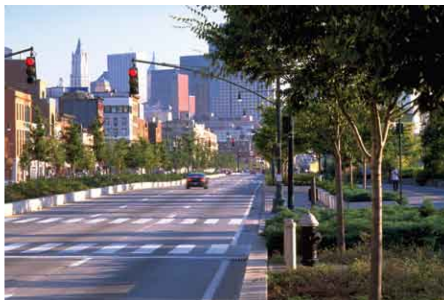
Manhattan's Greenwich Street (top) and Route 9A (bottom) have both been redesigned using high performance principles.
