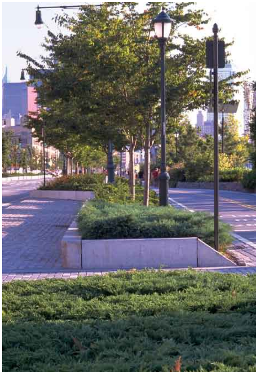
Route 9A Reconstruction – New York, NY
