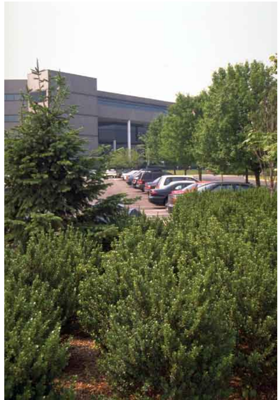
Prudential Insurance Company Headquarters – New Jersey Excavated site soil reused to create berms to screen parking lot
