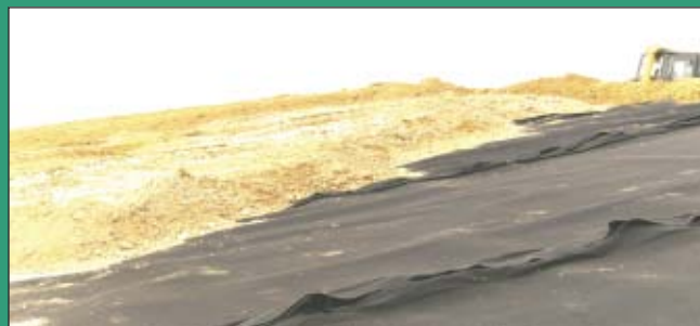
BARRIER PROTECTION MATERIAL OVER GEOCOMPOSITE
