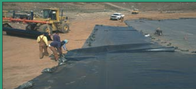
PLACEMENT OF GEOMEMBRANE
