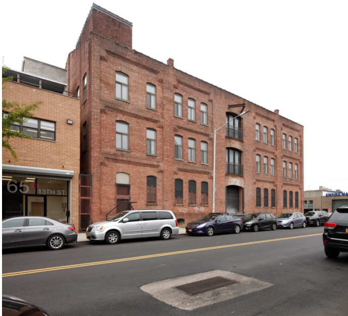
Montauk Paint Manufacturing Company Building (13th Street Facade) Sarah Moses, October 2019
