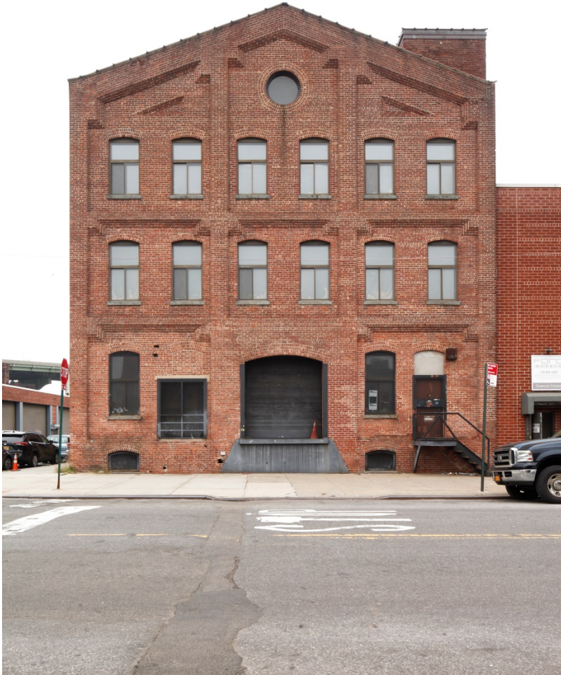
Montauk Paint Manufacturing Company Building (Second Avenue Facade) Sarah Moses, October 2019
