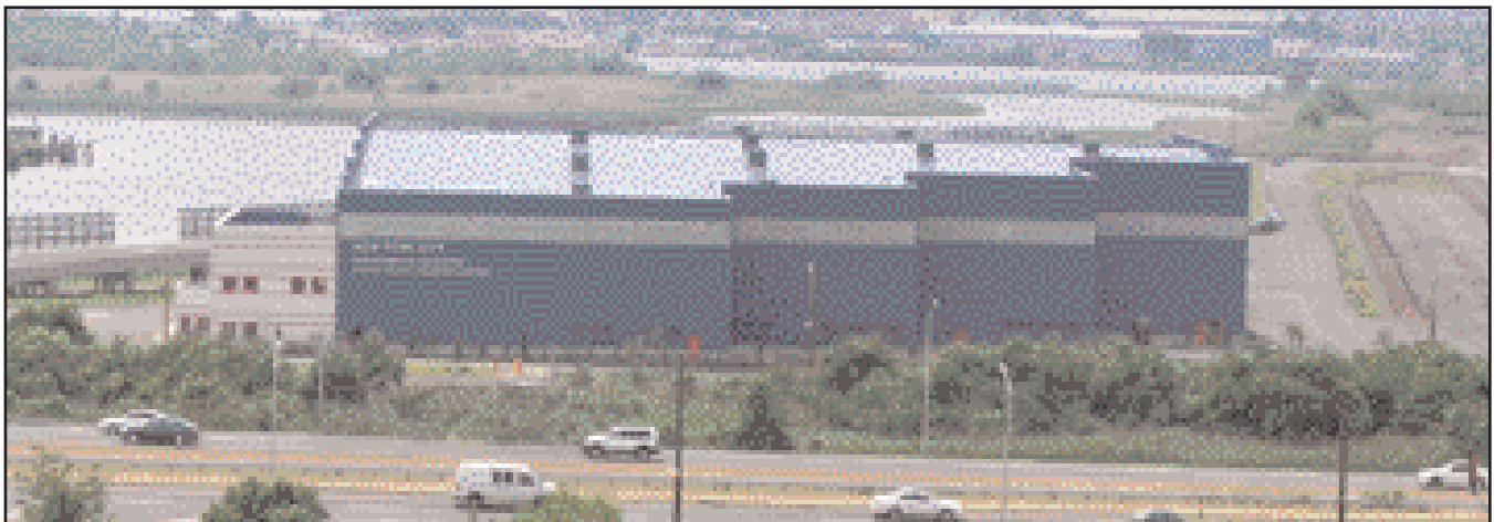
The new Staten Island Transfer Station
