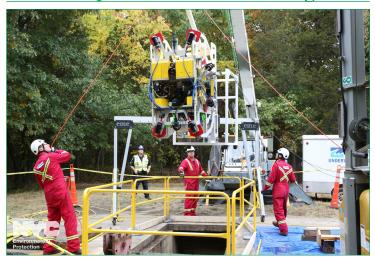
DEP <u>launched a remote operated vehicle</u> last week to pinpoint suspected leaks in a portion of the Catskill Aqueduct that runs several hundred feet below the Rondout Creek in Ulster County. The vehicle uses high-definition video cameras, acoustic equipment and other instrumentation to examine the interior of the aqueduct, known as the Rondout Pressure Tunnel. Data gathered through that analysis will be used to design any necessary repairs.
