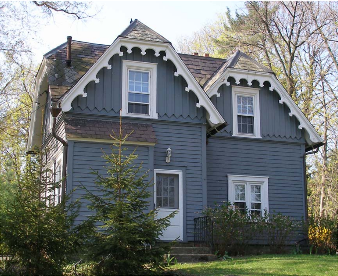
Greyston Gatehouse , east façade (upper) and north façade (lower)
