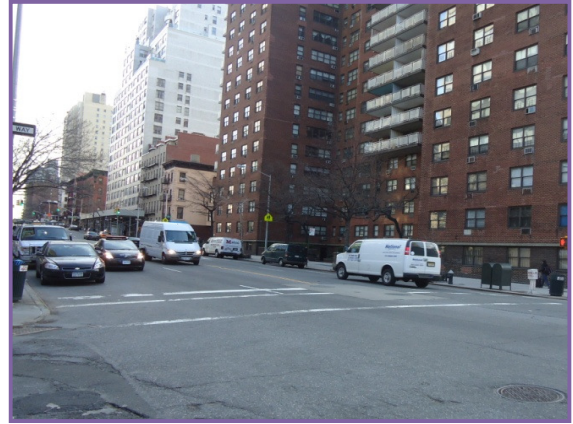
Photo No. 2: York Ave. & E 81 st St. (looking north)
