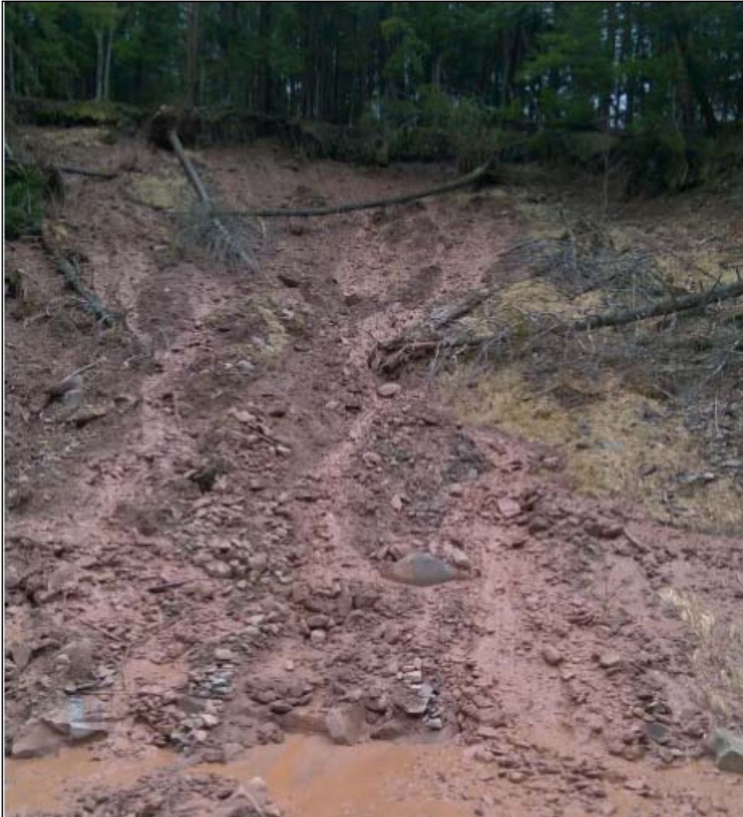
Figure 7. Example of hillslope failure at the Bull Run site.
