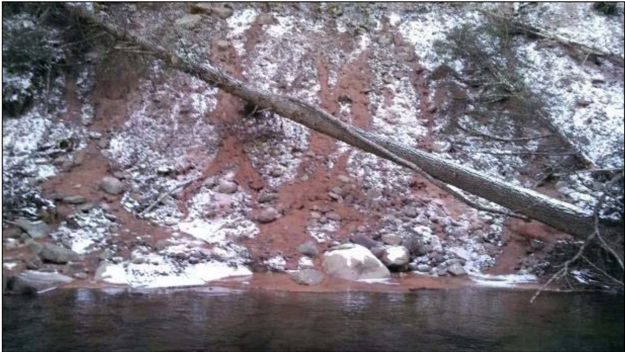
Figure 3. Example of freeze/thaw inducing turbid discharge from the hillslope.
