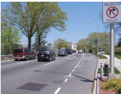
Whitestone Expressway NB Service Road -Looking south ➡
