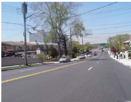
20th Avenue Looking West
