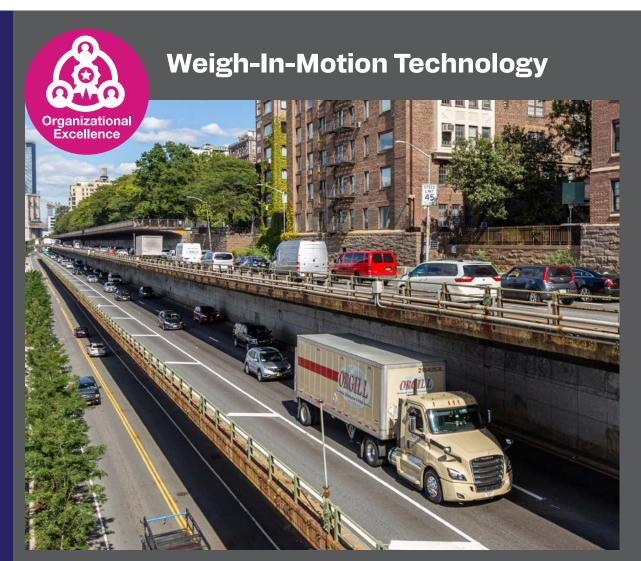
Bridge infrastructure is designed to last 50 to 100 years, with federal and state truck weight limits in place to ensure safety. However, with limited enforcement resources, many trucks are overweight, shortening the lifespan of bridges. With the use of weigh-in-motion (WIM) technology to automate enforcement of truck weights, NYC DOT can better protect the city's aging infrastructure.
