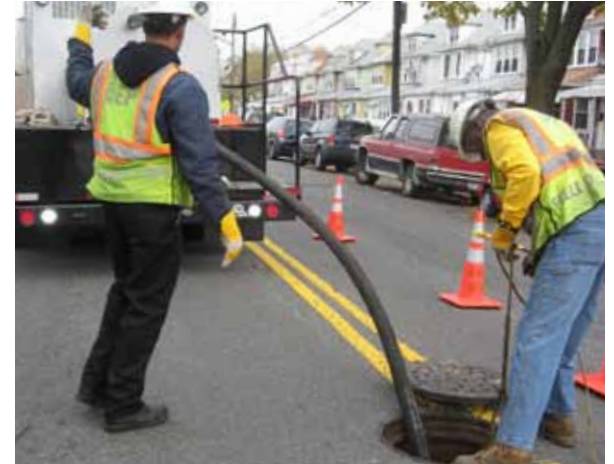
Mechanical rodders are used to clean accumulated grease and debris out of sewers. Rodders use a fast-moving rod to dislodge the debris from the sewer walls. The rod is at the end of a long, flexible hose that allows the machine to reach far into the line.
