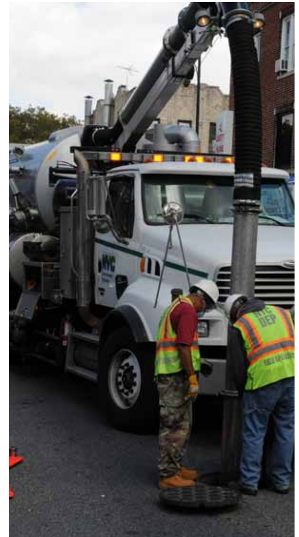
DEP crews use a Vactor truck to clean a sewer in Queens.
