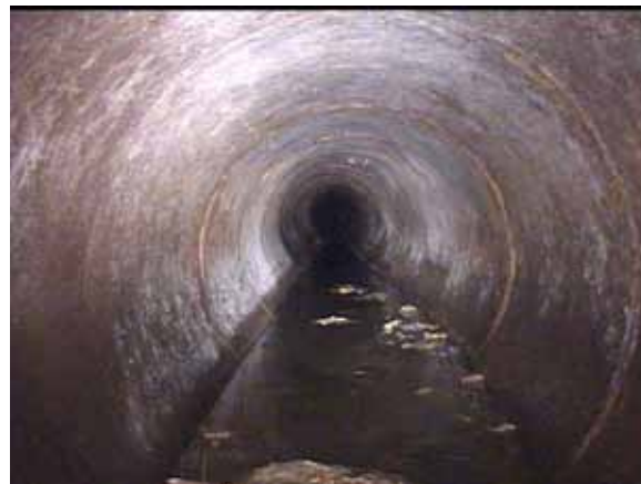
A clean sewer, without grease or oil build up, allows appropriate flow downstream.
