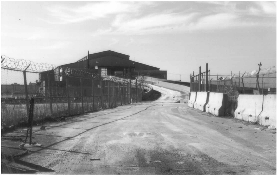
Figure 19.7-1 : View of the MTS building looking south from the site entrance. (Photo 2000)
