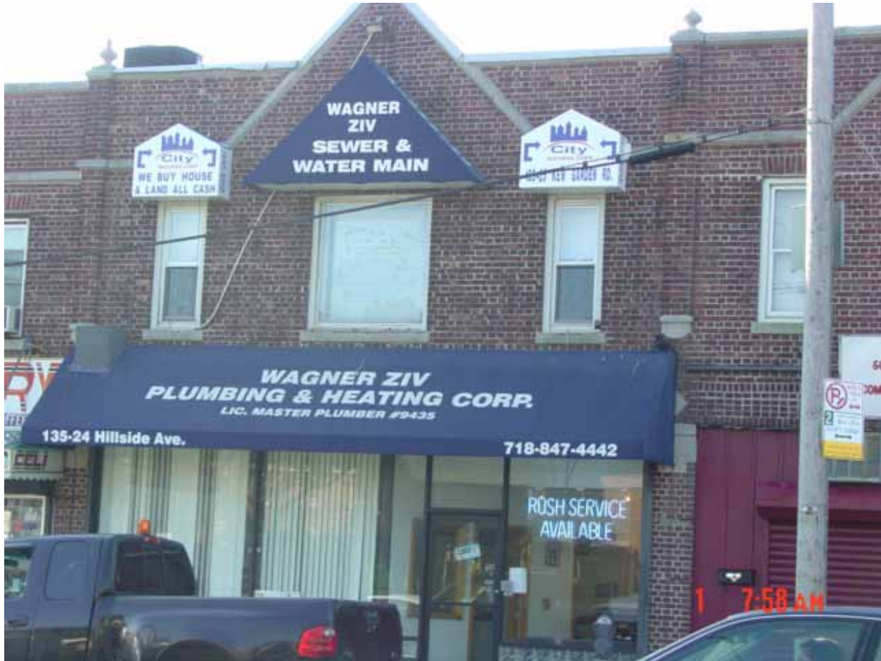
135-24 Hillside Avenue: Finance records inaccurately listed this property as “Primarily One-Family with One Store or Office” (Tax Class 1, Building Code S1).
