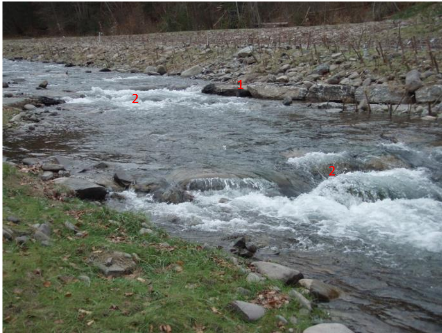
Figure 4.20 Stony Clove at Lanesville after restoration, showing heavy planting and bioengineering along far bank, and cross vane (1) with double sill (2).
