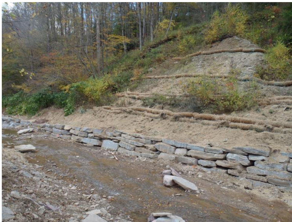
Figure 4.18 Third Brook, post-restoration, Slope #3, showing use of stacked rock wall to protect the toe of the slope with fascines, and coir logs to capture sheet erosion.
