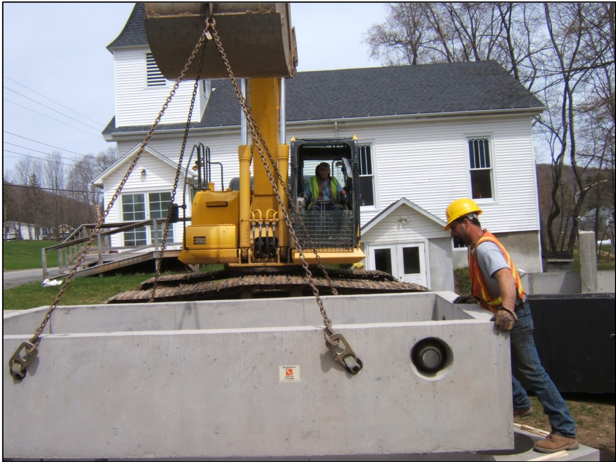
Figure 3.1 Installation of a grease trap as part of the Trout Creek CWMP project.
