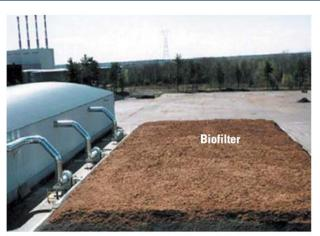
Photo 3-11: Conporec biofilter All process air from the receiving building, digester drum, and maturation building is filtered through a 200-by-80 foot biofilter.
