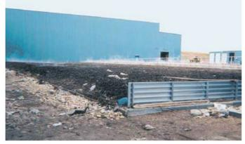
Photo 3-19: Biofilter at Edmonton facility Edmonton has three, above-ground, outdoor biofilters, which are composed of softwood bark and compost.
