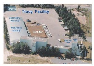
Photo 3-2: Aerial view of Conporec Tracy MSW-composting facility Located on a nine-acre site in the Tracy Industrial Park, the actual facility footprint is approximately two acres.
