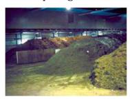
Photo 3-8: Inside Conporec maturation building The maturation building contains five concrete bays for maturing compost (primary screen unders).
