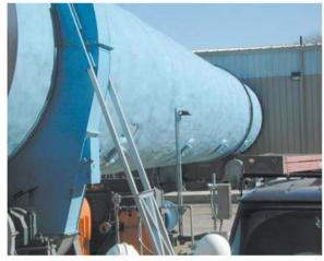
Photo 1-8: Digester Drum at the Marlborough Facility MSW loaded into the digester drum from the receiving building is discharged two to three days later in the air floor building.
