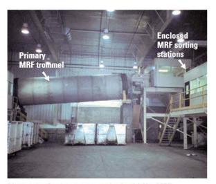
Photo 3-24: Sorting system at the Rapid City MRF
