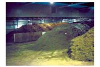
Photo 3-8: Inside Conporec maturation building The maturation building contains five concrete bays for maturing compost (primary screen unders).
