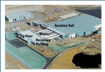
Photo 3-12: Aerial view of Edmonton facility The actual facility footprint is approximately 10 acres, which includes: receiving building, tip floor, five drums, primary screening area, aeration hall, refining area, biofilters, an office building, and parking.
