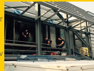
Workers Modifying SJU's HVAC System
