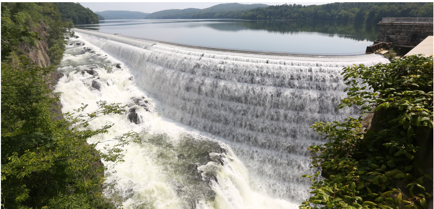
New Croton Dam Spilling
