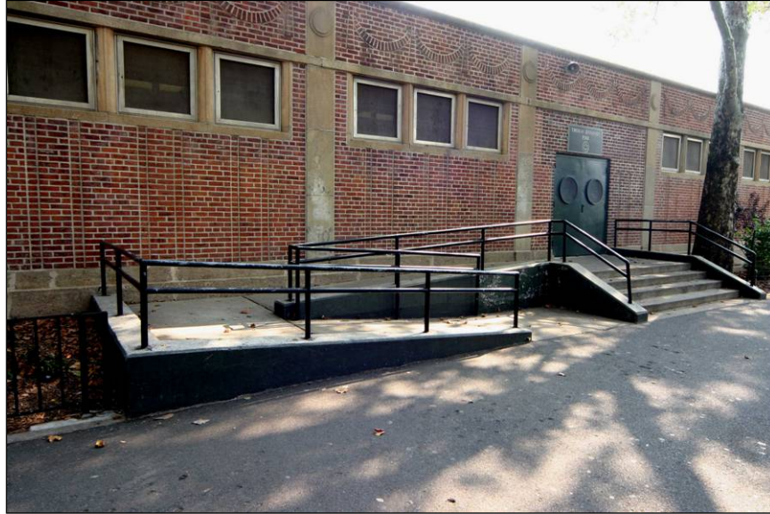
Thomas Jefferson Play Center: North Allee entrance ramp Photo: Carl Forster
