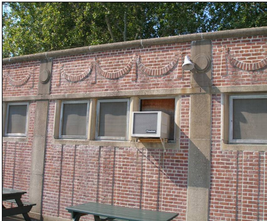
Thomas Jefferson Play Center: West Façade Photo: Theresa Noonan (Non-historic window air-conditioner with brackets, and Bull-horned speaker)
