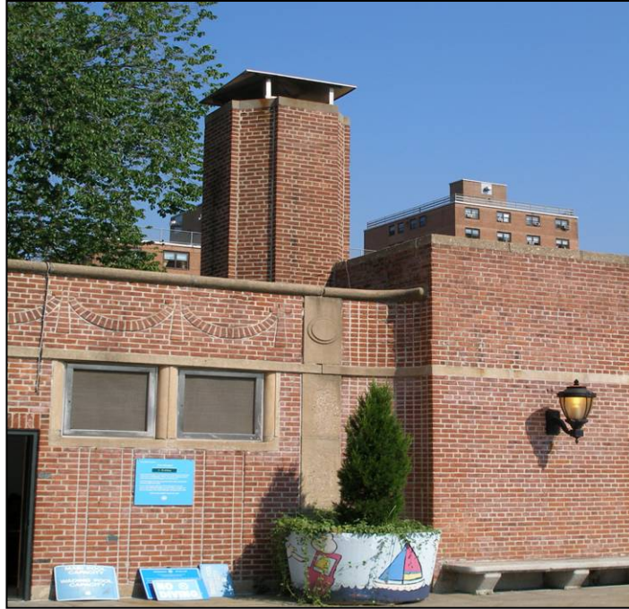
Thomas Jefferson Play Center: West Façade view of chimney Photo: Theresa Noonan
