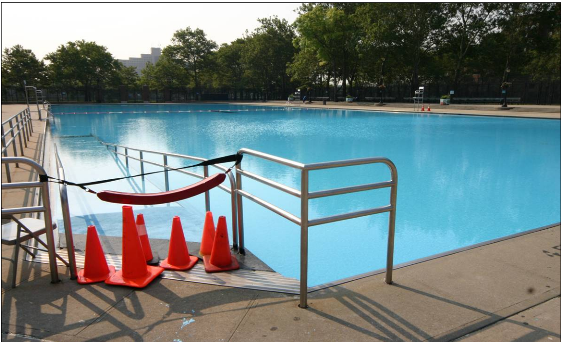
Thomas Jefferson Play Center: Pool Deck Area, main swimming pool (view southeast) Photo: Carl Forster
