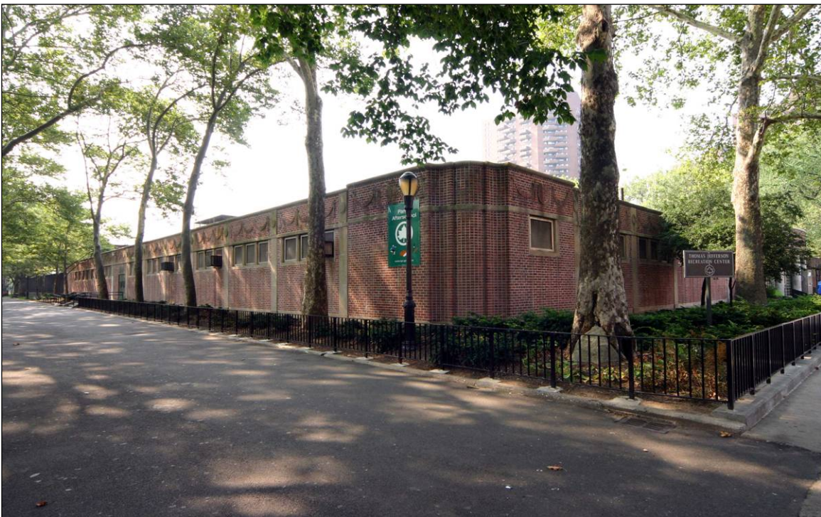
Thomas Jefferson Play Center: North Façade (view northeast) Photo: Carl Forster
