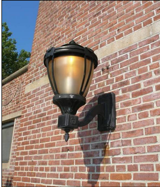
Thomas Jefferson Play Center: West Façade (non-historic sconce) Photo: Theresa Noonan
