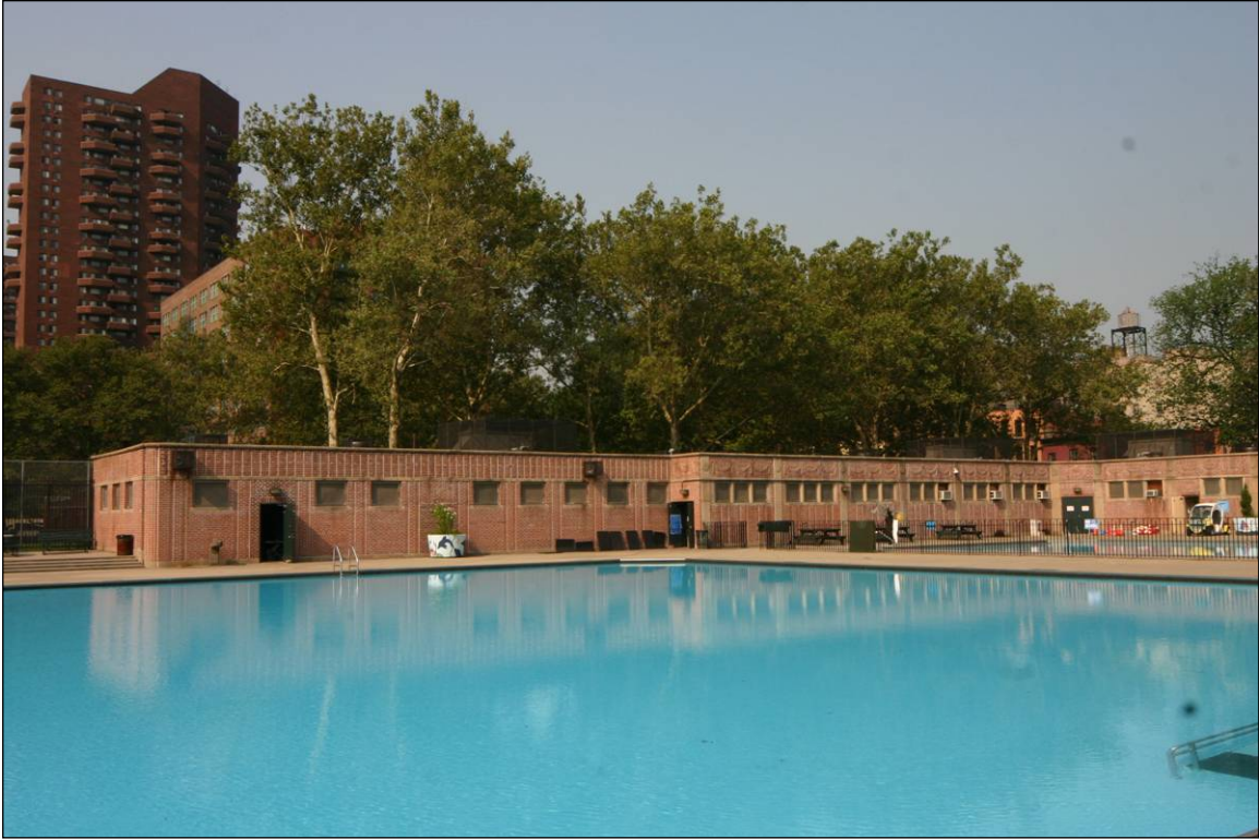
Thomas Jefferson Play Center: West Facade, south wing (view southwest) Photo: Carl Forster
