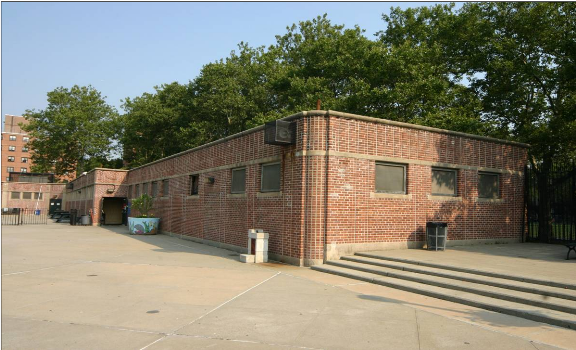
Thomas Jefferson Play Center: West Façade, North wing (view northwest) Photo: Carl Forster
