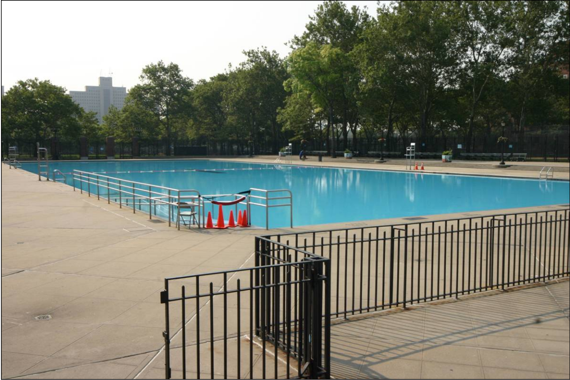
Thomas Jefferson Play Center: Pool Deck Area, main swimming pool (view southeast) Photo: Carl Forster
