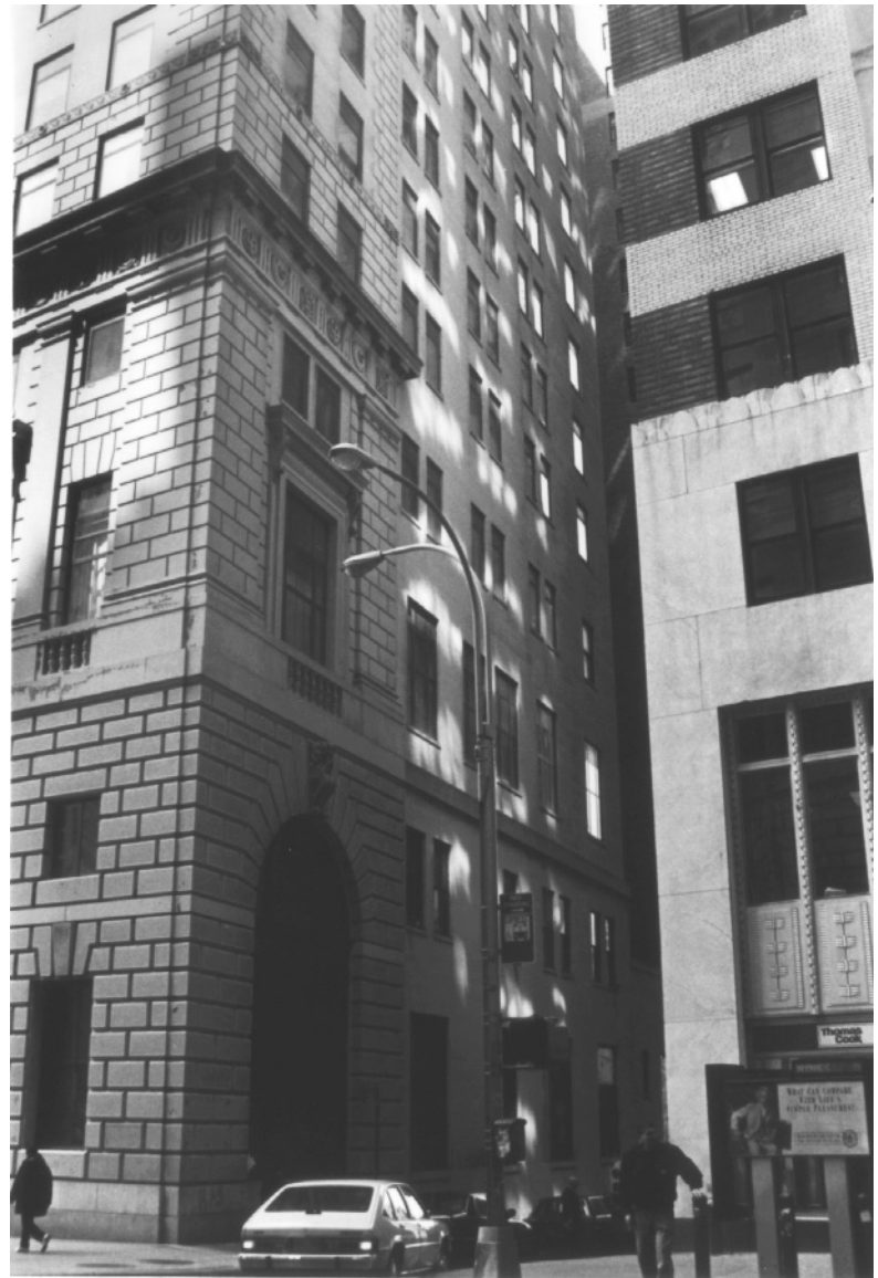
Fig. 5. Northwest corner of building and Morris Street elevation
