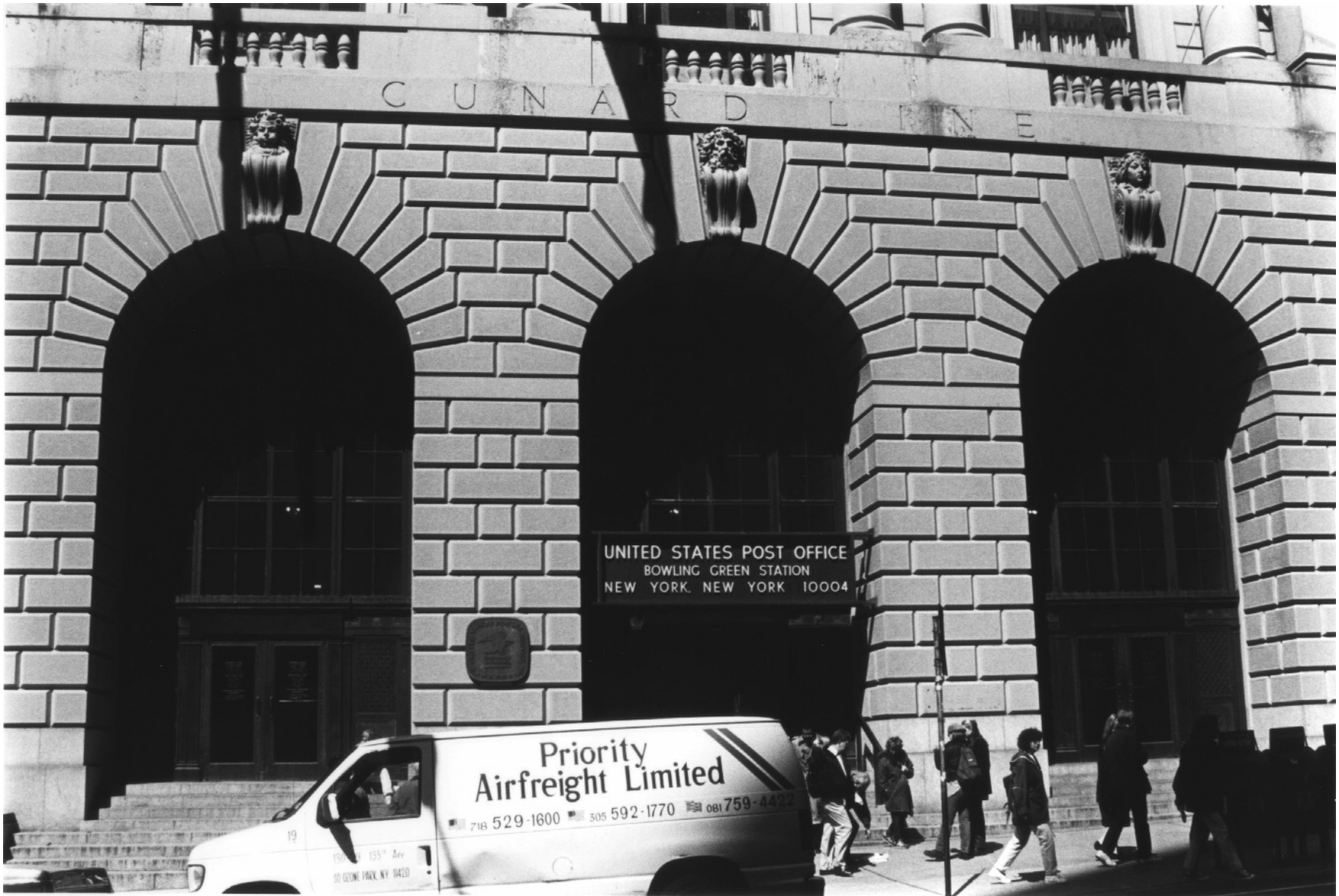
Fig. 3. Cunard Building, Detail of Broadway facade
