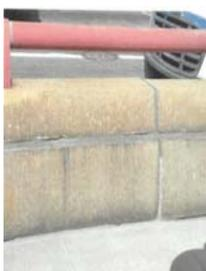
2019: Repointed Mortar at the Cap Stones and Joints of the Parapet Wall atop the Battery Park Underpass.
