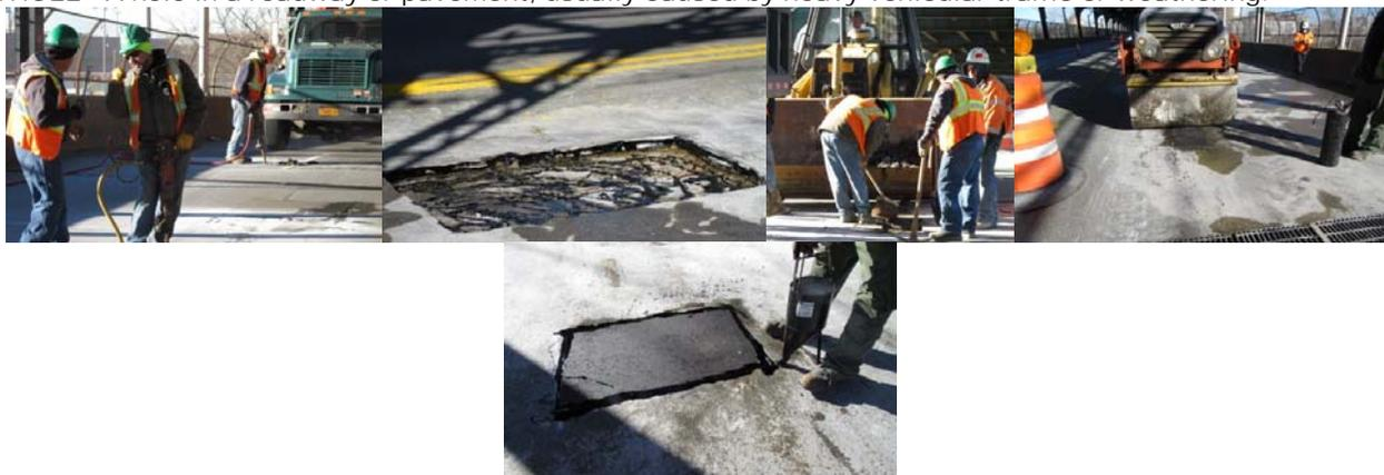
Repairing Potholes on the Roosevelt Avenue Bridge Deck Between Janet Place and 126th Street in January 2016. Each Perimeter is Sawcut. Filling in the Pothole With Asphalt. Paver Rolls Over the Pothole to Compact the Fill Material and Level the Surface. Finished Repair.
