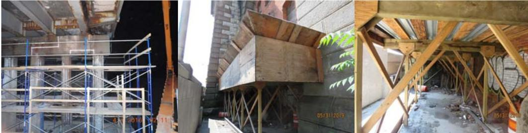
Old Mill Basin Bridge Scaffold Used During Pier Cap and Pier Column Repairs. 2019: Brooklyn Bridge Manhattan Approach, Arch Block A North Side - Overview of the Timber Scaffolding. View of the Underside of the Scaffolding.
