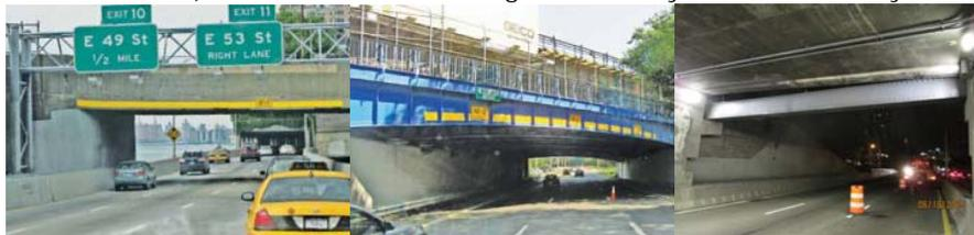
Retro-reflective Material Improves Visibility of These Low Vertical Clearance Bridges: East 60<sup>th</sup> Street Bridge over FDR Drive and Westchester Avenue Bridge over Hutchinson River Parkway. Vertical Clearance Beam at Span 53, Southbound Roadway of the Promenade over the FDR Drive. (FDR Credit: NYSDOT)
