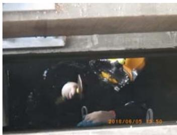
June 2018: Diver Installing a Splice Plate Underwater on the Belt Parkway over Gerritsen Inlet Bridge.
