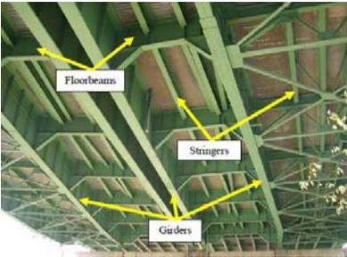
Steel Floor System and Main Supporting Members: Floorbeams, Stringers, and Girders. (Credit: FHWA Bridge Inspector’s Reference Manual)
