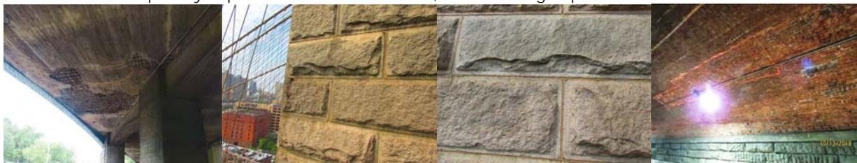
Hollow Sounding And Delaminated Concrete Areas With Exposed Rebars on the Sunrise Highway Bridge Westbound over Laurelton Parkway in 2014. Brooklyn Bridge Tower Stone Delamination in 2016. West Drive over Transverse Road #3 in 2018: Span 1 underside of arch near beginning abutment -Large area of scaled and delaminated brick facing area near begin abutment.
