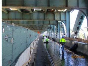
October 2018: Roosevelt Avenue Bascule Span - Bridge Deck Waterproofing Membrane Installation.
