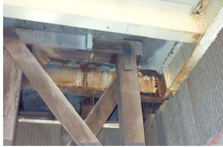
Timber Shoring Supporting a Failing Steel Beam – a Potential Winter Hazard. (Credit: Bojidar Yanev)
