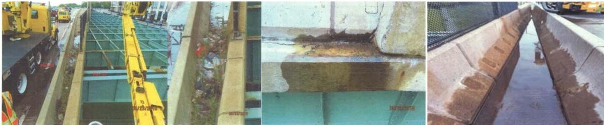
Safety Flag on the Miller Highway in 2018: Debris and Soil Accumulated Between the Jersey Barriers at Pier 55. This Caused Vegetation Growth and Water Ponding and Leaking Onto the Girders. This Leads to Pavement Deterioration and Girder Rust. The Debris and Soil Were Removed.
