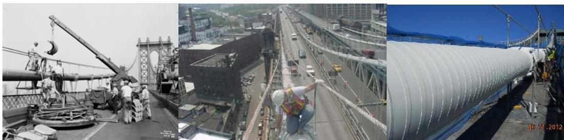
Replacing Cables on the Manhattan Bridge in 1955. (Credit: NYC Records) Inspector on Manhattan Bridge Cable. Cable B. (Credit: NYSDOT)
