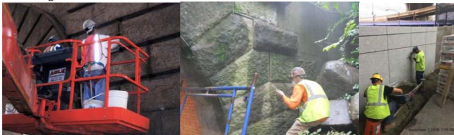
Pointing Joints on the East Face of the Brooklyn Anchorage of the Manhattan Bridge. Pointing the Masonry on the East Drive Bridge (East Wood Arch). 2018: Brooklyn Bridge Contract #6 - Ramp I - Pointing Joints.
