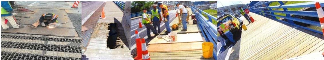
Union Street Bridge over Gowanus Canal –Straightened, Cleaned, Ground, and Welded Roadway Plate #5 on Span #4 in 2019. Safety Flag: Borden Avenue Bridge over Dutch Kills – Broken Wooden Planks of the Right Sidewalk at Span #1.
