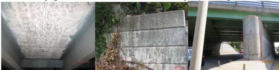
Union Street Bridge over Brooklyn-Queens Expressway in 2012 – Extensive Map Cracking With Efflorescence on the Underside of the Deck. (Credit: NYSDOT) Tompkins Avenue Bridge over B&O Railroad (Abandoned) in 2016 - Map Cracks With Efflorescence Near the End of the Wing Wall. Hamilton Place Bridge over Long Island Expressway in 2019 – Pier 1, Left Face of Stem.
