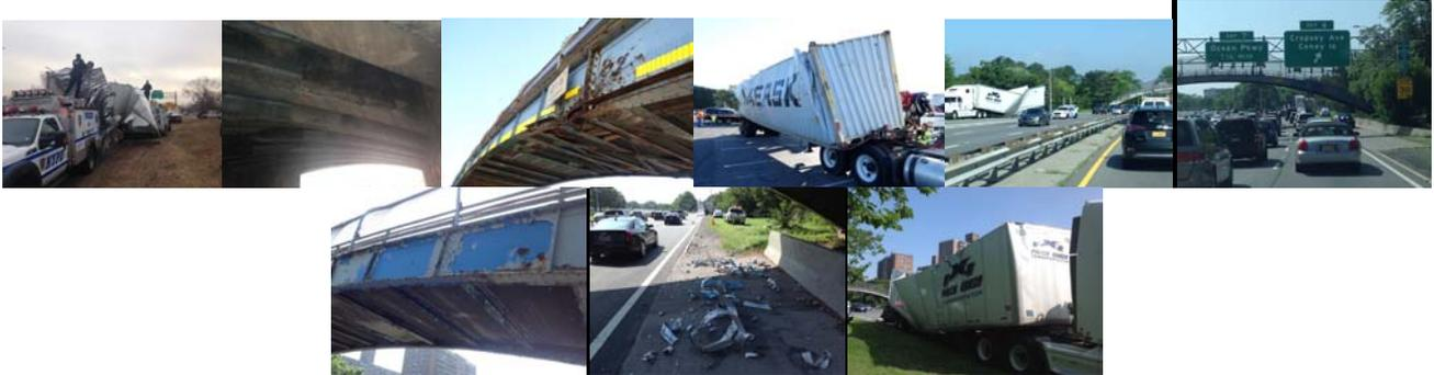
Douglaston Parkway Bridge Strike in 2015: Police Observing the Truck Damage. Underside of Bridge Concrete Beams Only Exhibited Scratches. (Credit: Artemio Angeles) 17<sup>th</sup> Avenue Pedestrian Bridge Strike in 2015. 27<sup>th</sup> Avenue Pedestrian Bridge Strike in 2018 – Truck, Bridge, and Debris.
