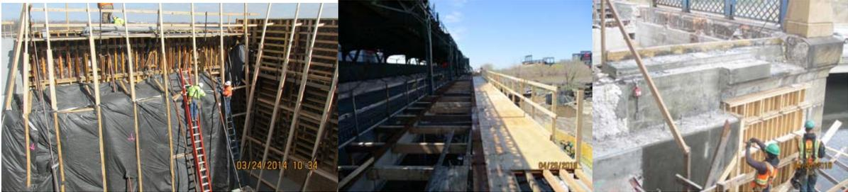
Gerritsen Inlet Bridge in March 2014: Putting up Insulated Forms in Preparation for the Placement of Concrete at the West Abutment Wingwall. The Insulation Helps Protect the Concrete From the Elements and Fluctuating
