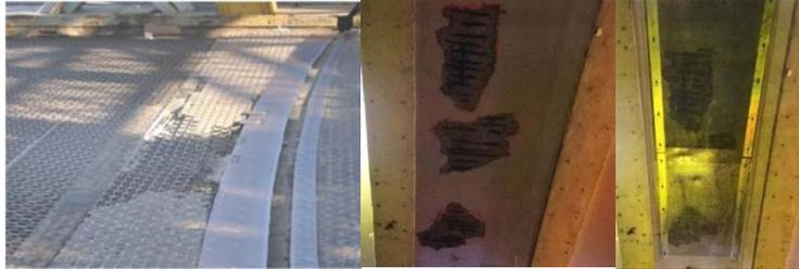
Example of PIA Safety Flag: Broken Grating. Chipping and Shielding at the Park Avenue Viaduct. Crew Removed Loose Concrete and Installed Expanded Sheet Metal Protective Shielding on the Underside of the Deck at Span #6.
