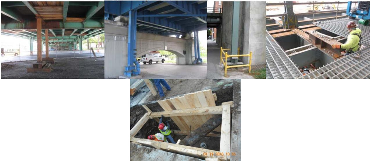
2014: Timber Shoring at Spans 7 and 8 of the Harlem River Drive over Ramp to and From Northbound Harlem River Drive. 2016: Steel Shoring at Span 5 of the East 174<sup>th</sup> Street Bridge over the Sheridan Expressway. Eastbound Brooklyn-Queens Expressway over Washington Street – Shoring on the Right Side of the End Abutment. 2018: Roosevelt Avenue West Viaduct Span 10 – Shoring for Steel Column Repairs, and Forest Avenue Culvert over Crystal Avenue - Installed Timber Shoring and Sheeting.
