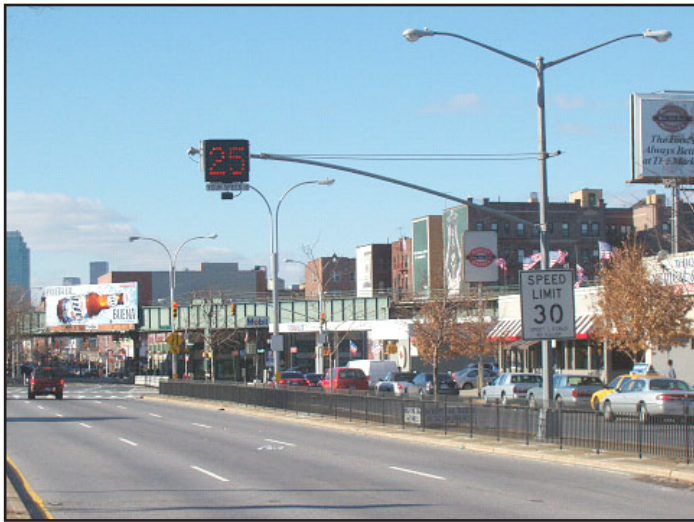
Example of permanently mounted speed detector board to inform motorists of their travel speed
