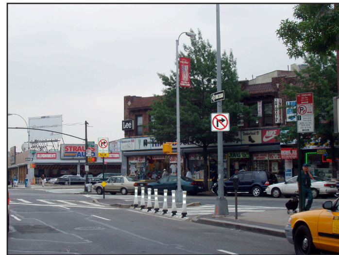
Signage and flexible bollards were used as temporary treatments to eliminate the uncontrolled right turn onto Greenpoint Avenue
