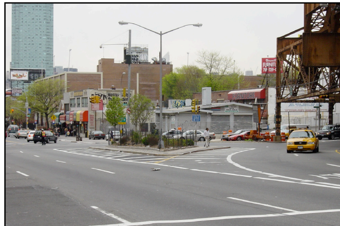
Channelization and markings at the convergence of Queens Boulevard, Van Dam Street and Thomson Avenue
