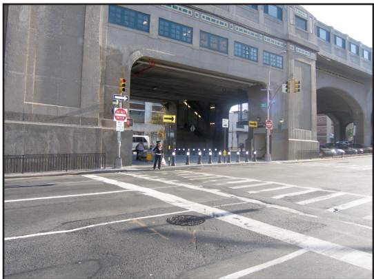
Detailed images and perspectives of full closure of 33 rd Street, including signage, reflective bollards, pedestrian fencing and the protected pedestrian plaza
