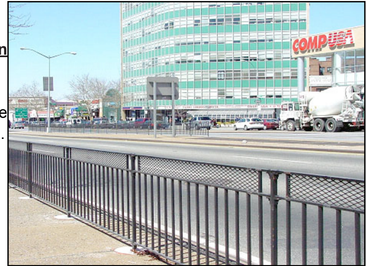
Pedestrian fencing along Queens Boulevard
