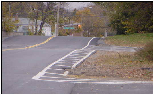
Roadway markings were utilized to improve geometry of roadway, narrow the roadway into one travel lane and provide parking
