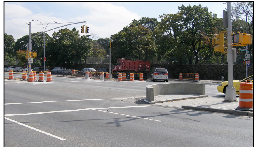
Median extensions and concrete protection devices being constructed along Queens Boulevard
