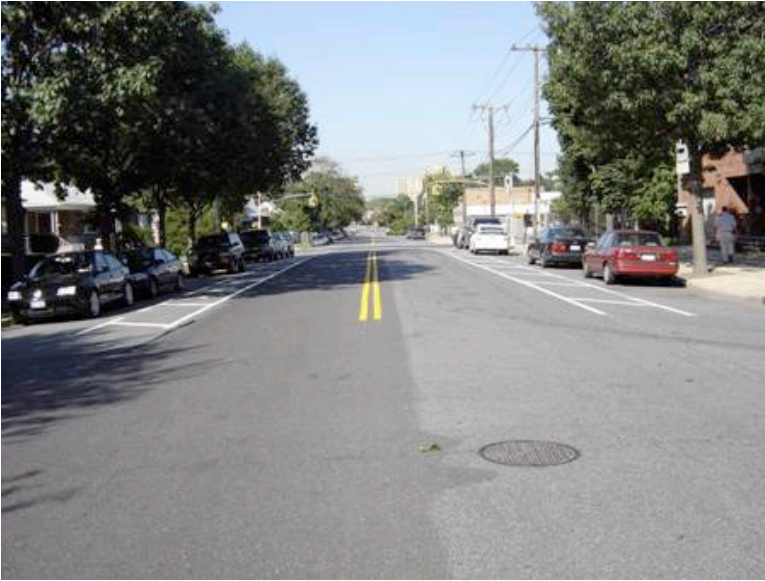
Roadway markings effectively narrowed 80 th Avenue to one lane in each direction
