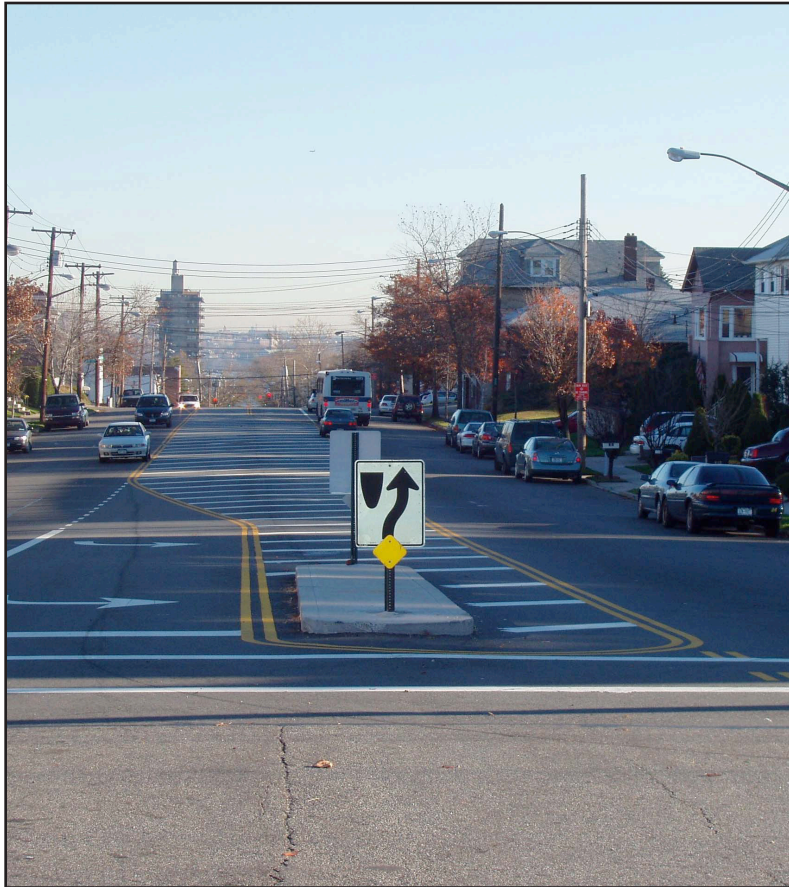
Roadway markings and raised intersection at the Hylan Boulevard and Reynolds Street
