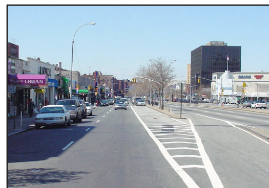
Top: Pavement Marking advising pedestrians to “Wait for Walk Signal”. Middle : Example of parking along the center median. This strategy narrowed the roadway to one lane from two. Bottom: At some locations, parking meters were removed and roadway markings and flexible bollards were installed to improve vehicular and pedestrian safety.
