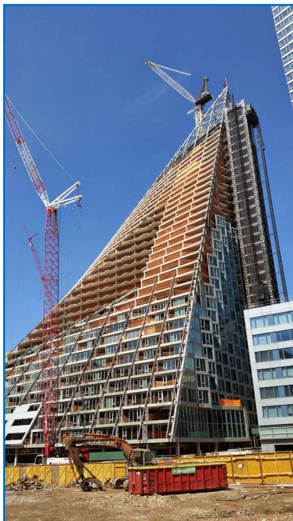
Figure 6: The cascading roofline on this OER E-designated site in Manhattan optimizes the sun exposure for maximum passive lighting potential.
