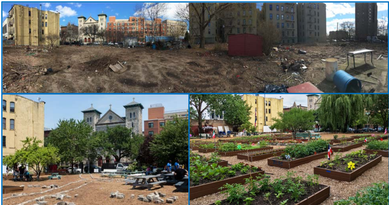
Figure 7: The NYC Clean Soil Bank was able to provide capping for a garden in the Bronx that limited exposure to potentially contaminated historic fill, and laid the foundation for the addition of raised beds.
