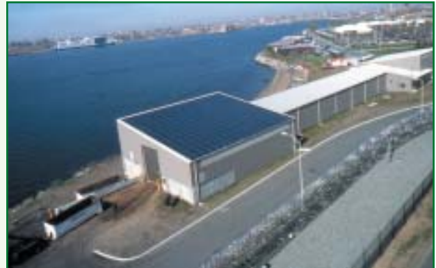
Aerial view of Riker’s Island and the in-vessel, food-waste-composting facility. The facility features the world’s largest installation of a translucent photovoltaic panel roofing system. Installed with funding from the New York Power Authority, the roof panels provide 40 kilowatts of power to the plant.
