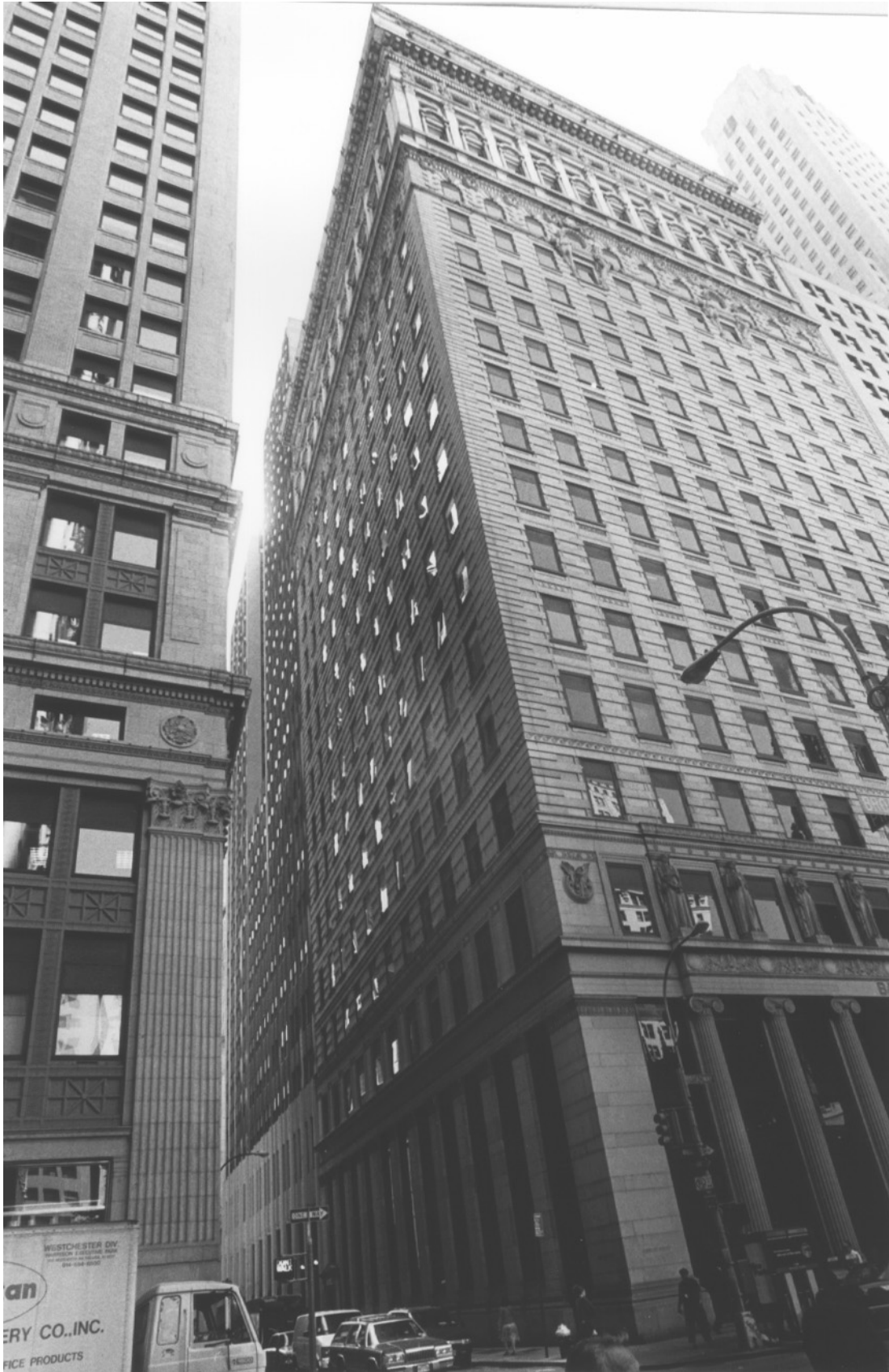
American Surety Building 100 Broadway, Manhattan View from the northwest showing Pine Street and Broadway facades Photo: Carl Forster
