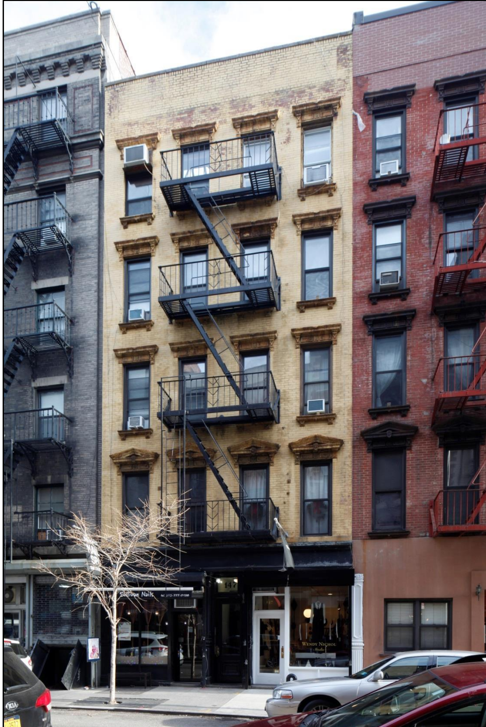
Figure 12 147 Sullivan Street (Architect A.H. Blankenstein, Owner John Rabenstein, built 1875) Photo: Sarah Moses, 2016
