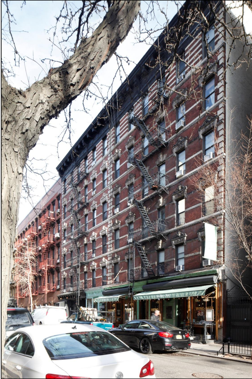
Figure 21 137 Sullivan Street (left) and 135 Sullivan Street (right) (Architect Horenburger & Straub, Owner Isaac Grossman and Michael Charles, built 1904) Photo: Sarah Moses, 2016
