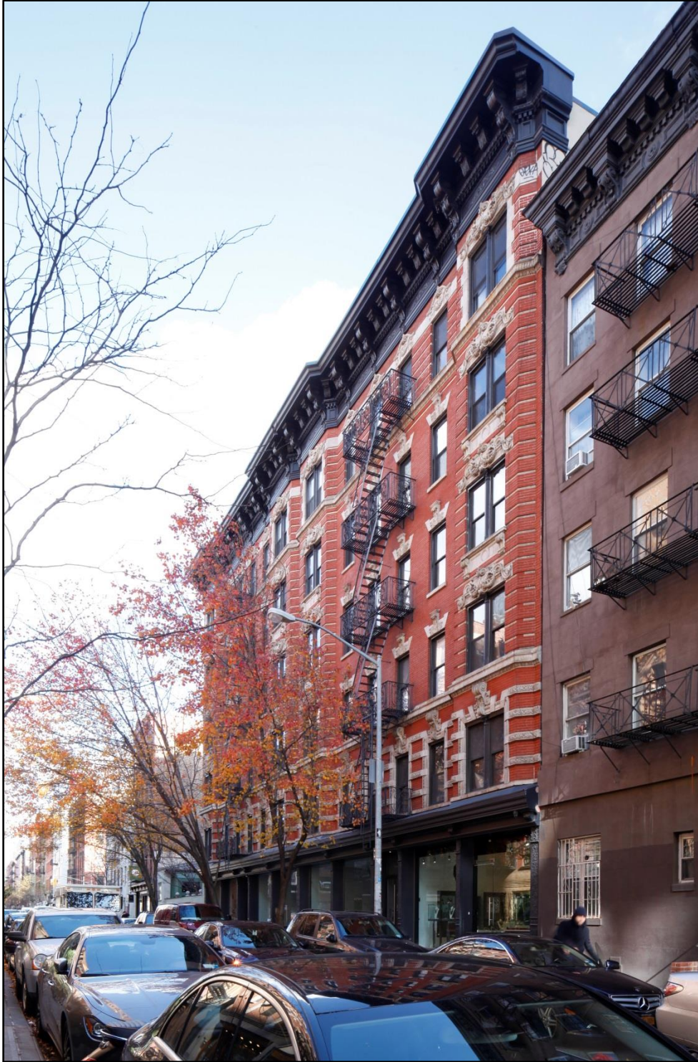
Figure 28 68 Thompson Street (right) and 72 Thompson Street (left) (Architect John Hauser, Owner Soloman Jacobs, built 1904) Photo: Sarah Moses, 2016
