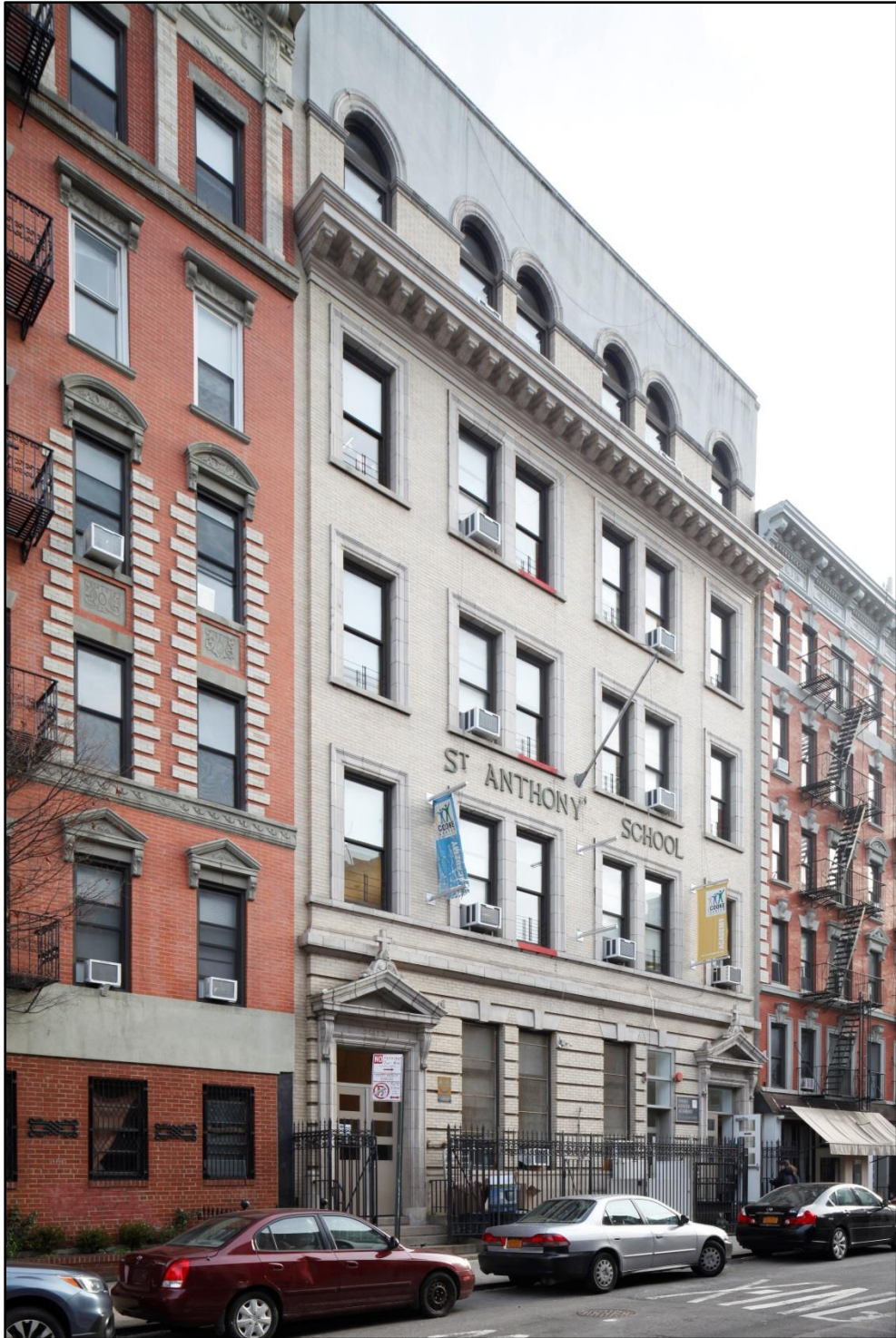
Figure 37 60 MacDougal Street St. Anthony's School (Architect Nicholas Serracino, Owner St. Anthony of Padua Roman Catholic Church, built 1909) Photo: Sarah Moses, 2016
