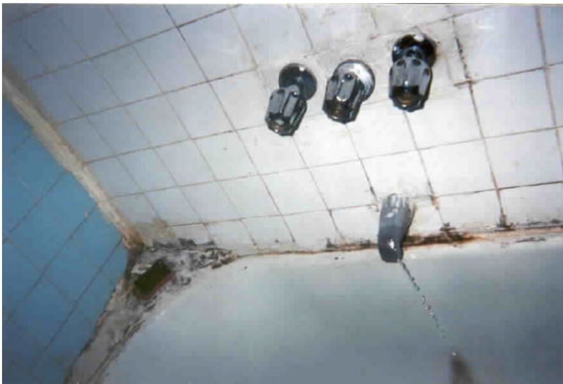
Apt. #5A - Picture 11 - Faucet leaks and mold in bathroom
