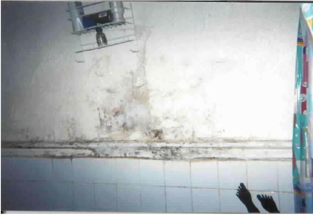
Apt. #5A - Picture 11 - Faucet leaks and mold in bathroom
