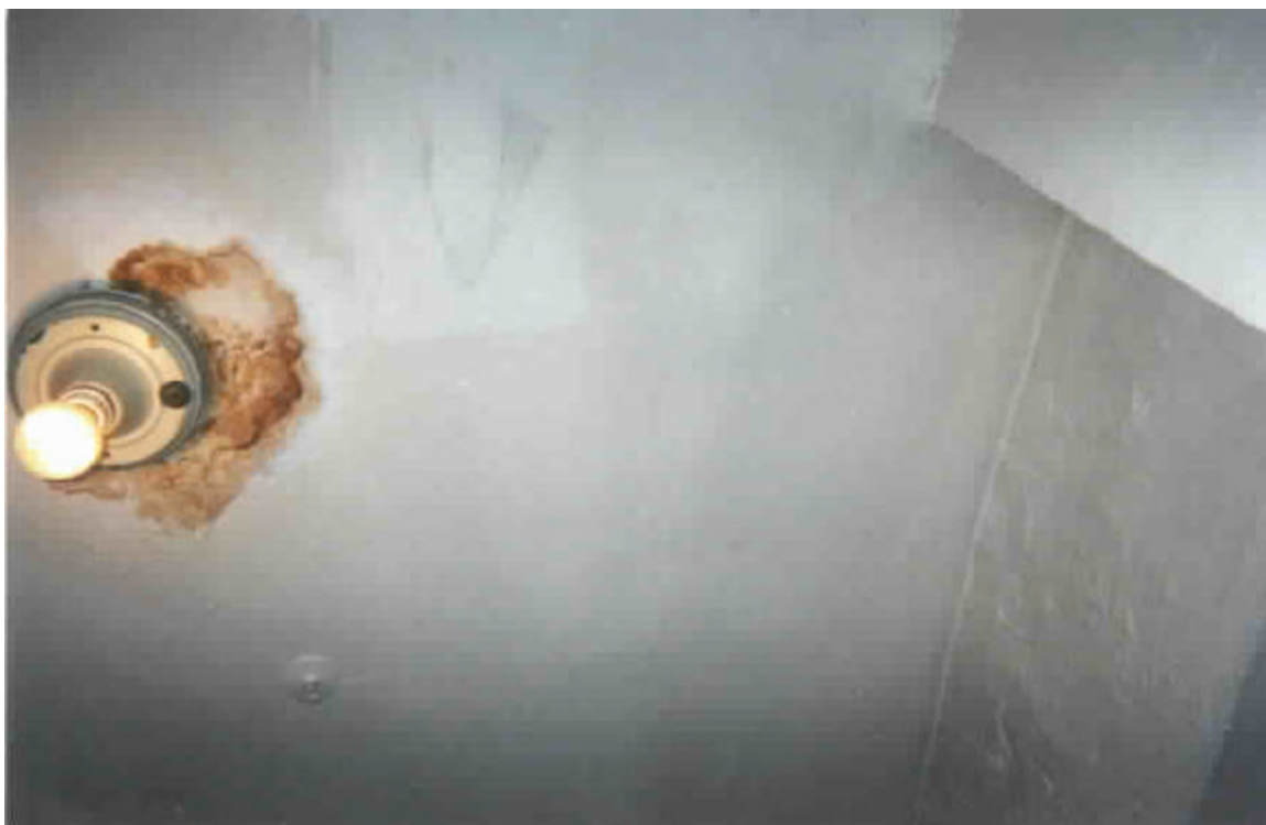
██████████ Apt. 2B - Picture #2 - Leak next to kitchen light
