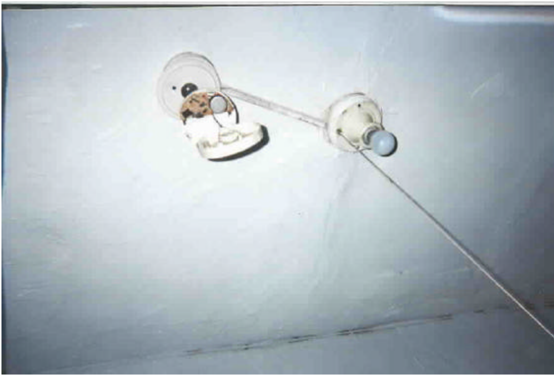
Apt. 21 - Picture #6 - Smoke detector hanging off ceiling
