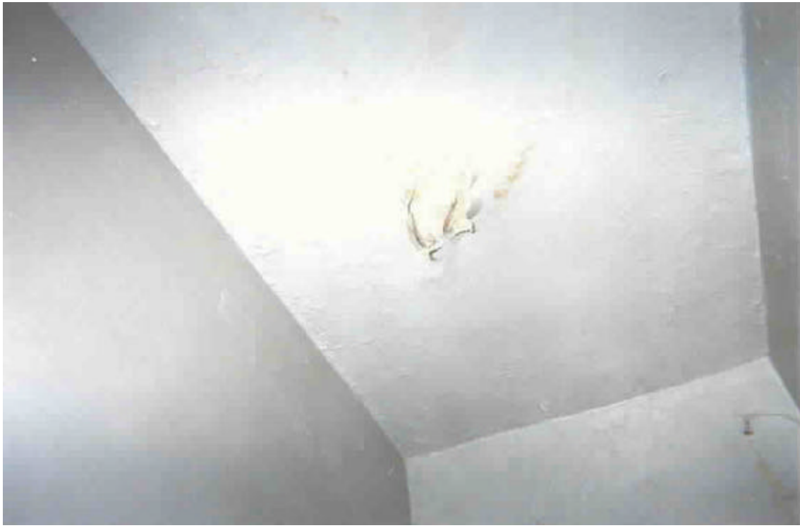
██████████ Apt. 2B - Picture #2 - Leak next to kitchen light
