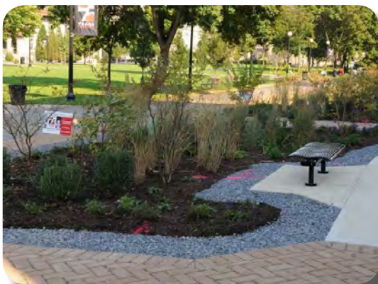
Green infrastructure in parks used to treat stormwater at its source.
