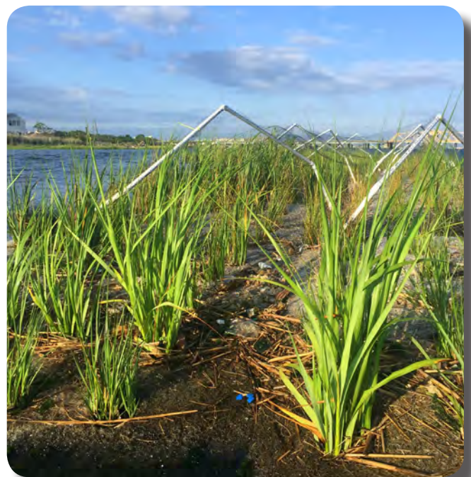
Floating “wetland” wave attenuator.
