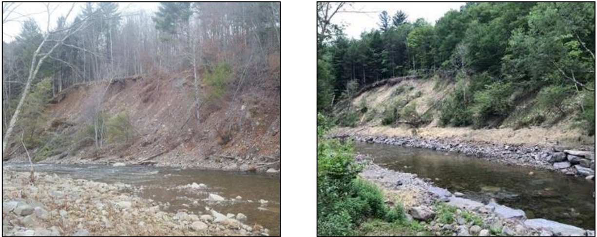
Figure 4. Denning Town Hall Streambank Stabilization – before (left) and after (right).
