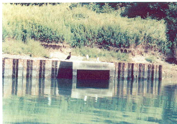
Storm sewer outfall in Fresh Creek Photograph: L. Kachalsky, O'Brien & Gere
