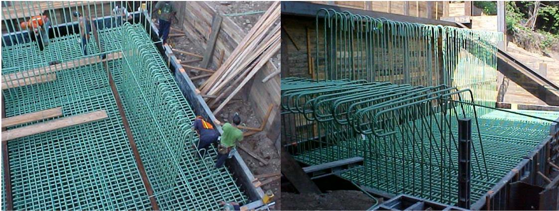
Installation of Abutment Footing and Stem Reinforcement for the 14<sup>th</sup> Avenue Bridge
