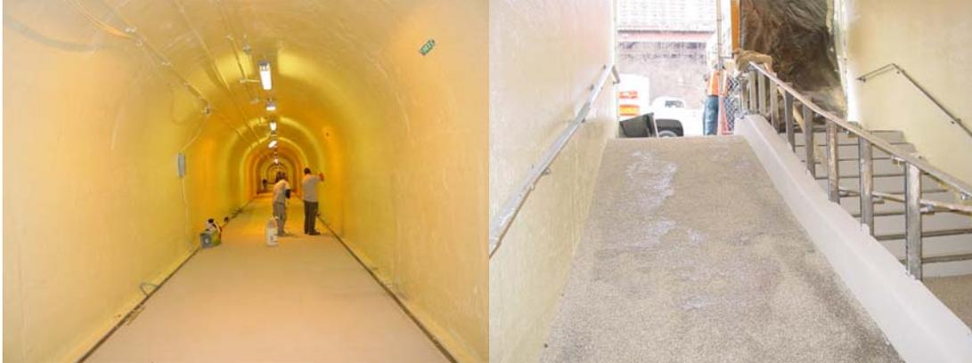
Applying the 2<sup>nd</sup> Skid Resistant Coating to the Western Half of the Tunnel Floor. Repaired Staircase With a Skid Resistant Coating on the Ramp and Landing. (Credit: Thomas Leung)
