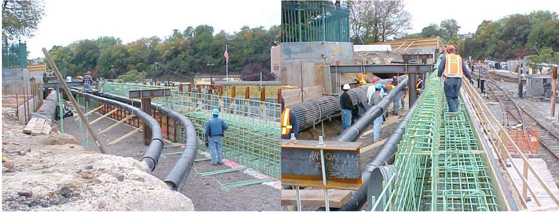
Installation of Reinforcement in the 7<sup>th</sup> Avenue Bridge Abutment Stem and Backwall
