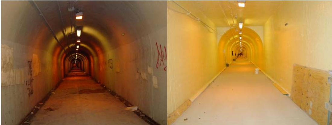
Western Half of 191<sup>st</sup> Street Tunnel Before Repairs and Painting. Repairs Almost Completed – the Tunnel's Lighting Creates the Yellow Tint. (Credit: Thomas Leung)
