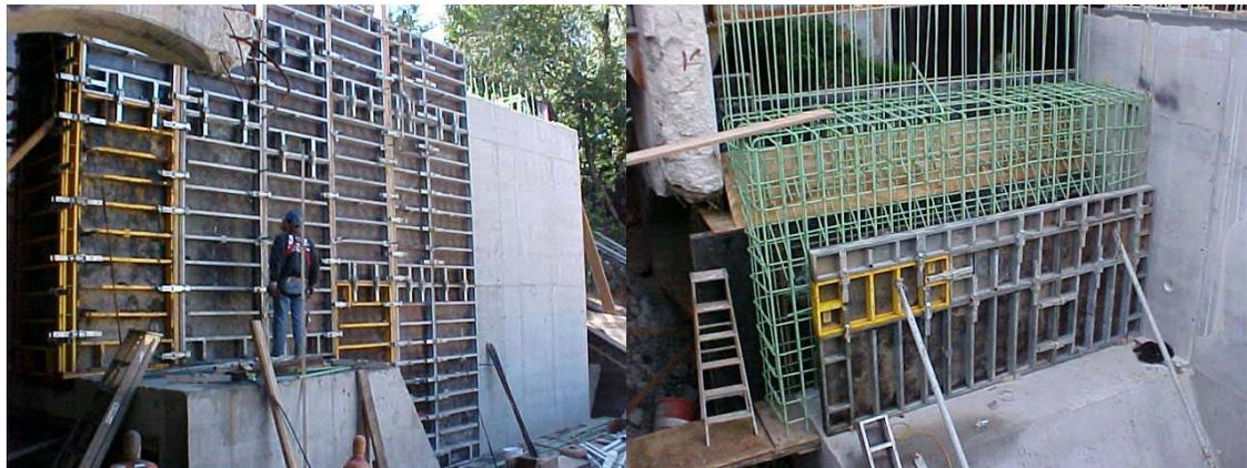
View of Reinforcement and Form Work Installation at the 14<sup>th</sup> Avenue Bridge Abutment
