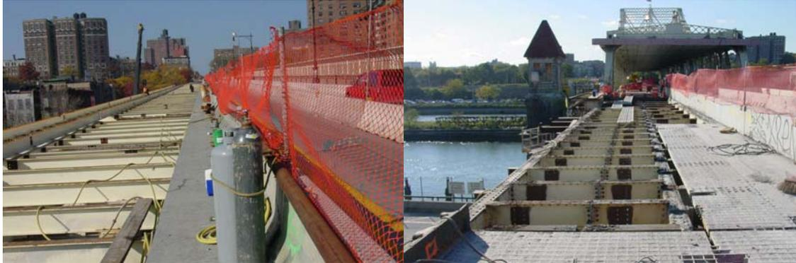
Looking West Along the West 155<sup>th</sup> Street Viaduct of the Macombs Dam Bridge. Demolition of Truss Deck.
