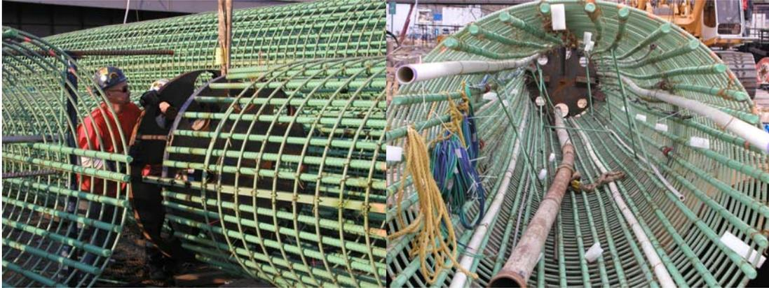
Osterberg Load Cell and Bearing Plate at Bottom of Reinforcing Cage. Instrumentation, Integrity Testing Tubes, And Concrete Tremie Pipe Within A Completed Reinforcement Cage.
