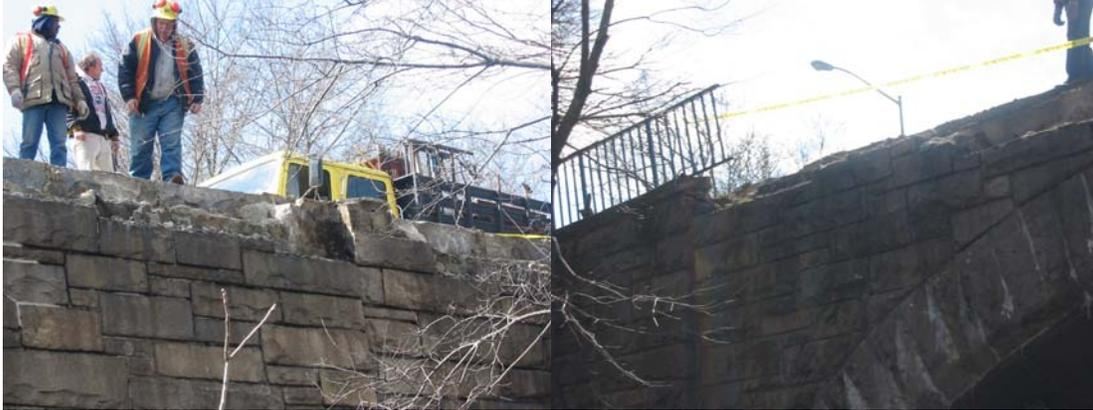
A Multi-Vehicle Accident Resulted in Damage to the Stone Cladding and About 200 Feet of Bridge Rail.
