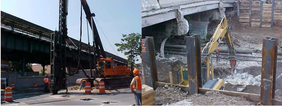
Installation of the Soldier Piles for the Excavation Protection System for the 14<sup>th</sup> Avenue Bridge. Excavation for the Abutment Footing.
