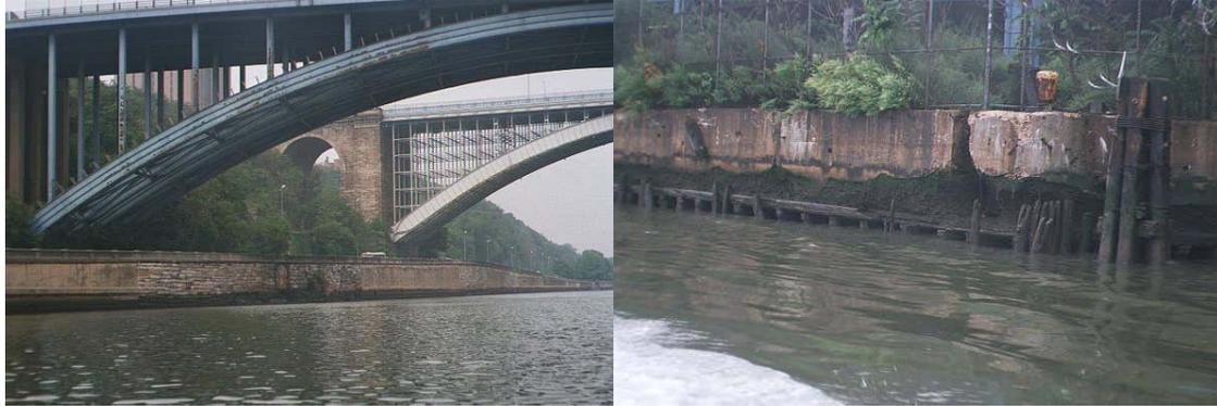
Bulkhead at Alexander Hamilton Bridge. Severe Erosion of the Concrete Seawall Allowing Loss of Fill at the MTA Rail Yard at 151<sup>st</sup> Street.
