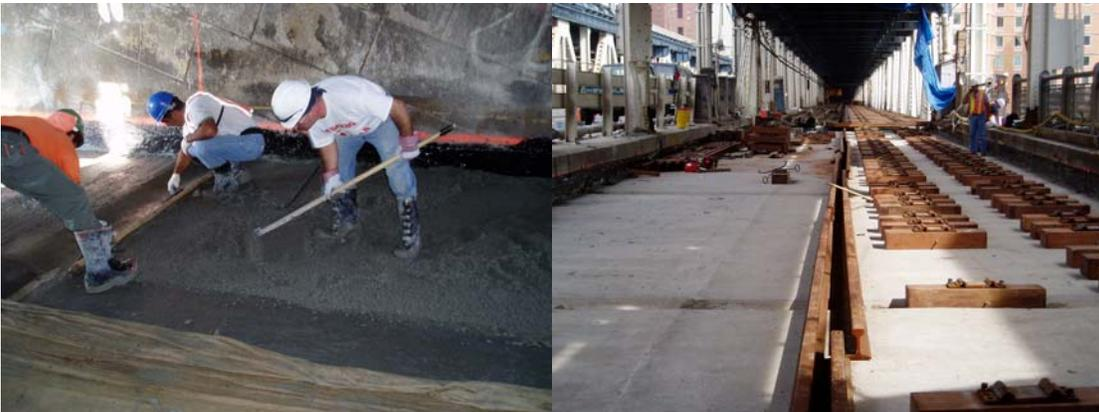
Placing the Waterproof Protection Layer on the Anchorage Roof Inside the North Track Envelope.
