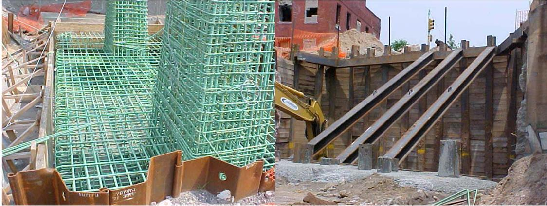
Installation of Footing and Column Reinforcement for the 2<sup>nd</sup> Avenue Bridge's Center Pier. Excavation Protection System at the North Abutment.
