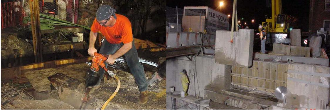
Exposing the Old Steel Stringer Ends on the 91<sup>st</sup> Place Bridge. Removing the Central Pier by Saw Cutting the Concrete in Two Directions – Each Piece Weighed 9 Tons.
