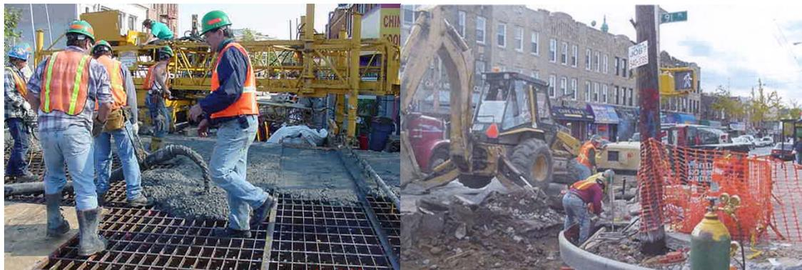
Placing Concrete for the 91<sup>st</sup> Place Bridge Grid Deck. Installation of New Sidewalk and Roadway at the Corner of Corona Boulevard and 91<sup>st</sup> Place.
