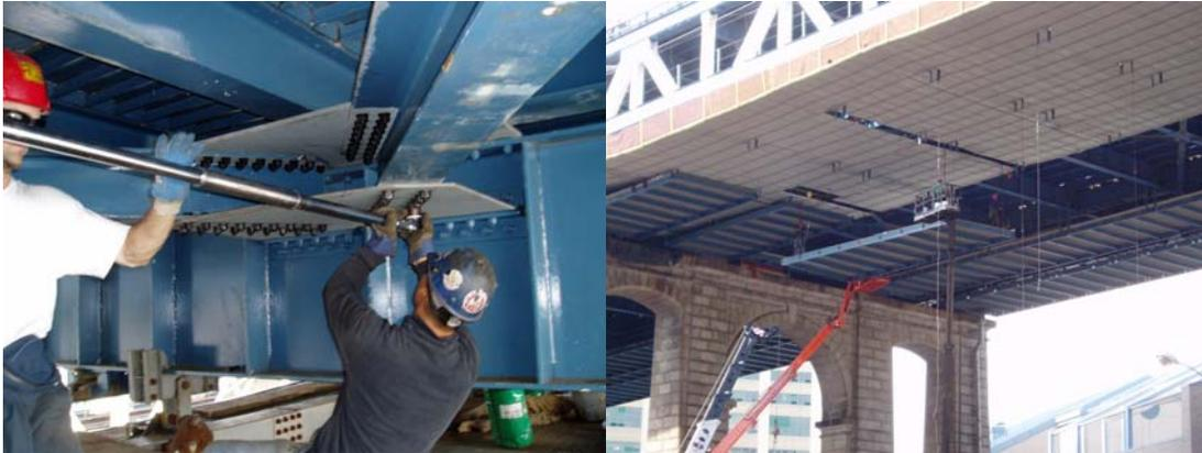
Torquing the Bolts for the Installation of the Upper Laterals for the Truss Stiffening System.
