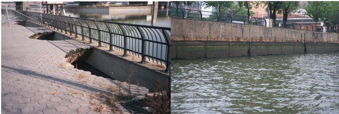
Severe Pavement Undermining and Collapse at 145<sup>th</sup> Street Due to Fill Loss Through Corroded Steel Sheet Piling. East River Bulkhead.
