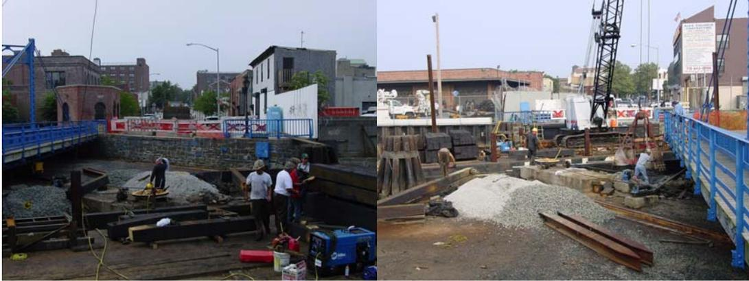
Cutting 12x12 Timbers On the Barge to Match the Wall. Clam Bucket Used for the Backfilling Operation at the Carroll Street Bridge. (Credit: Thomas Leung)
