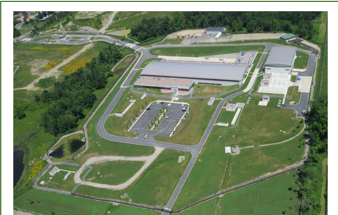
Figure 4.12 Aerial photo of the Catskill/Delaware Ultraviolet Disinfection Facility, the largest of its kind in the world.
