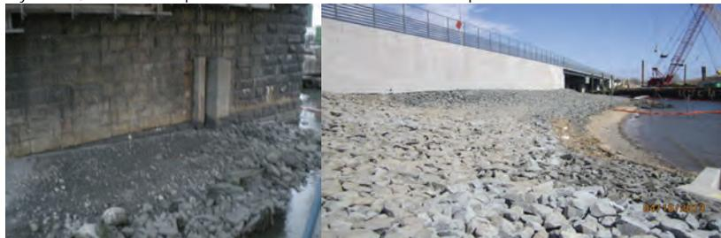
Eroded Riprap Pier Protection at Pier 11 of Old Willis Avenue Bridge in 2008. (Credit: NYSDOT) Riprap Installed in 2013 on South Side of Belt Parkway Bridge over Fresh Creek, Facing East.
