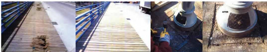
May 2015 Safety Flag: Borden Avenue Bridge Over Dutch Kills - Wooden Planks of Sidewalk Damaged After Vehicle Accident. East 14<sup>th</sup> Street Bridge Over LIRR Bay Ridge –Ironworkers Fabricated and Installed the Bottom Cover of the Ventilation Post on the Right Sidewalk.
