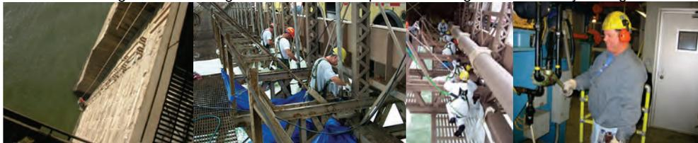
Repairing the Brooklyn Bridge Standpipe System, 130 Feet Below the Roadway. Maintenance Crew Conducting the Annual Cleaning and Lubrication of the Solid Rod Suspenders and Spherical Bearings on the Brooklyn Bridge. 2<sup>nd</sup> Photo - Oilers Steven Marxhausen, Rene Francis, Richard Morreale, Thomas McAuliffe, and Andrew Sorrentino. (Credit: Anatoly Orlov) Oiler T. McAuliffe at the 9<sup>th</sup> Street Bridge
