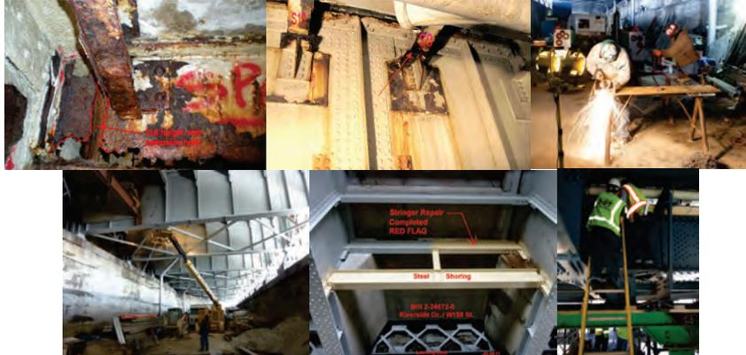
September 2008: Advanced Corrosion of Steel Stringer and Girder. February 2011: Red Flag Stringer Repair at Riverside Drive Viaduct over West 158<sup>th</sup> Street. July 2015: Assistant Civil Engineers Andrew Hoang and Clara Medina Inspecting a Red Flag on the Manhattan Bridge From the Motorized Bridge Inspection Traveler Platform Beneath the Bridge.
