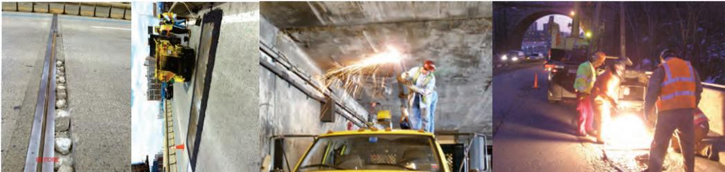
August 2014 PIA Safety Flag: Broken Joint Concrete Header And Steel Armor on the Long Island Expressway over Dutch Kills Creek. The Condition Was Made Safe By Installing Two Steel Plates. PIA Flag (Truck Wedged Under the FDR Drive at Span 41): Removing the Debris. (Credit: Victor Sandoval) PIA Flag Repair (Through Hole) on Harlem River Drive Ramp. (Credit: Bojidar Yanev)
