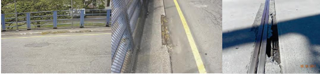
Spalled Section of Curb on the East 8<sup>th</sup> Street Bridge in 2006. (Credit: NYSDOT) Spalling With Exposed Rebar on the Beginning Abutment Joint Header of the Westchester Avenue Bridge over the Bronx River in 2011.
