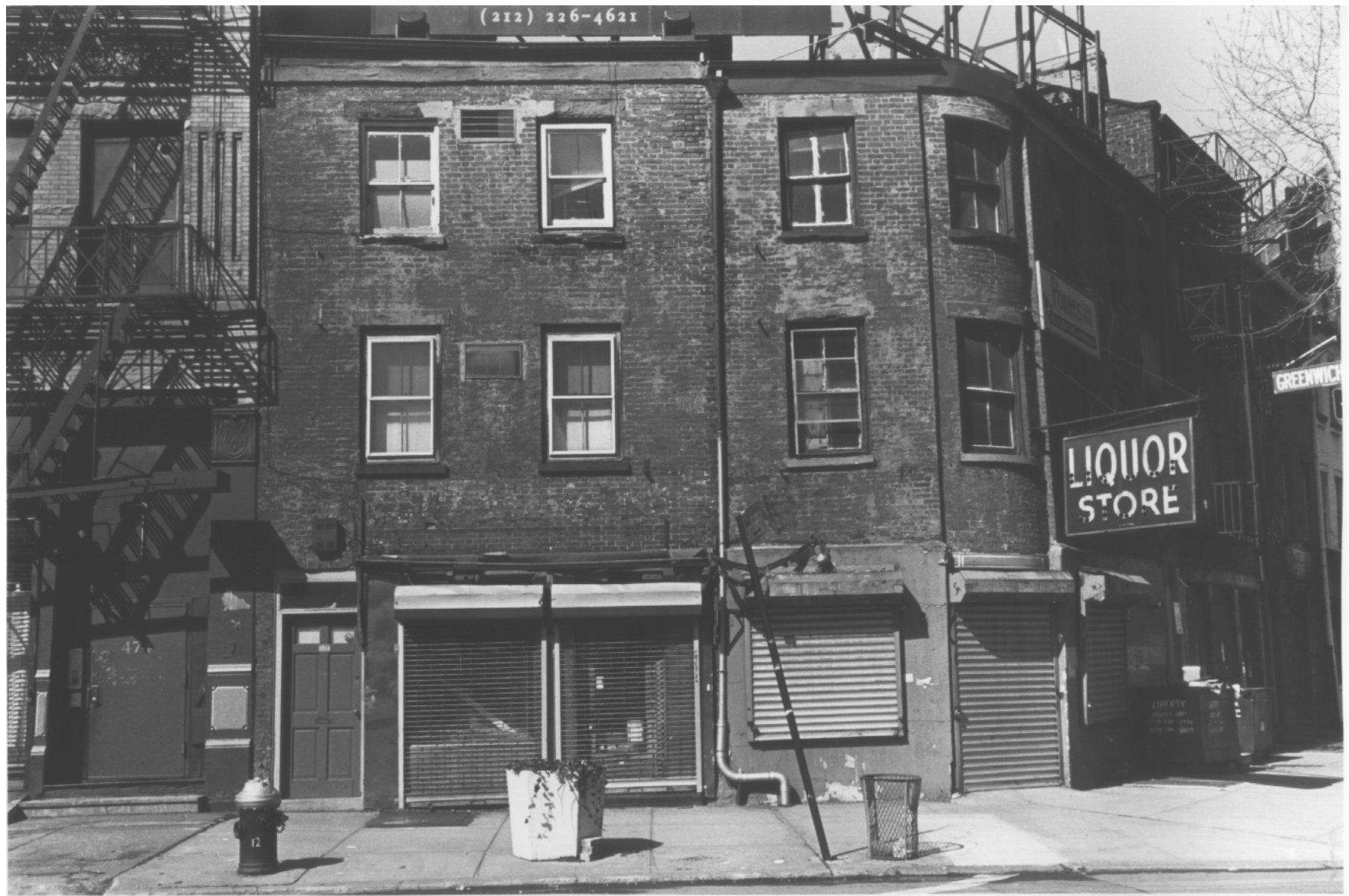
480 Greenwich Street/502 Canal Street House, Manhattan Greenwich Street facade Photo: Carl Forster , March 1988
