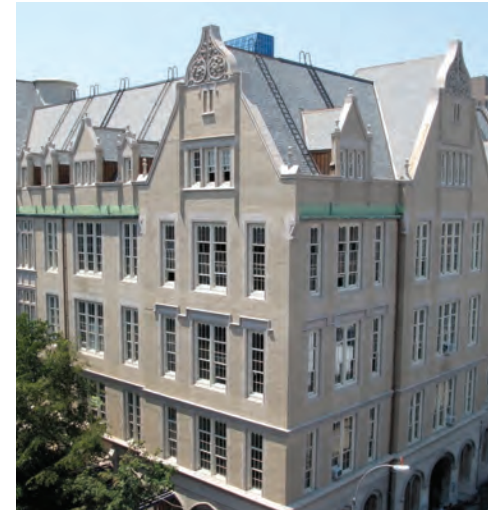
Clemente Soto Velez Cultural & Educational Center renovated façade, Manhattan
